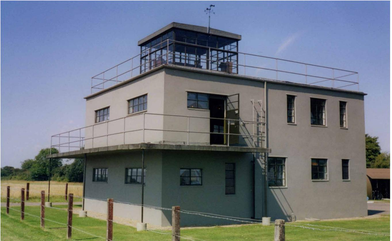
Watch tower at Thorpe Abbots (Norfolk) following restoration in which the original windows were refurbished and the glass house rebuilt.
