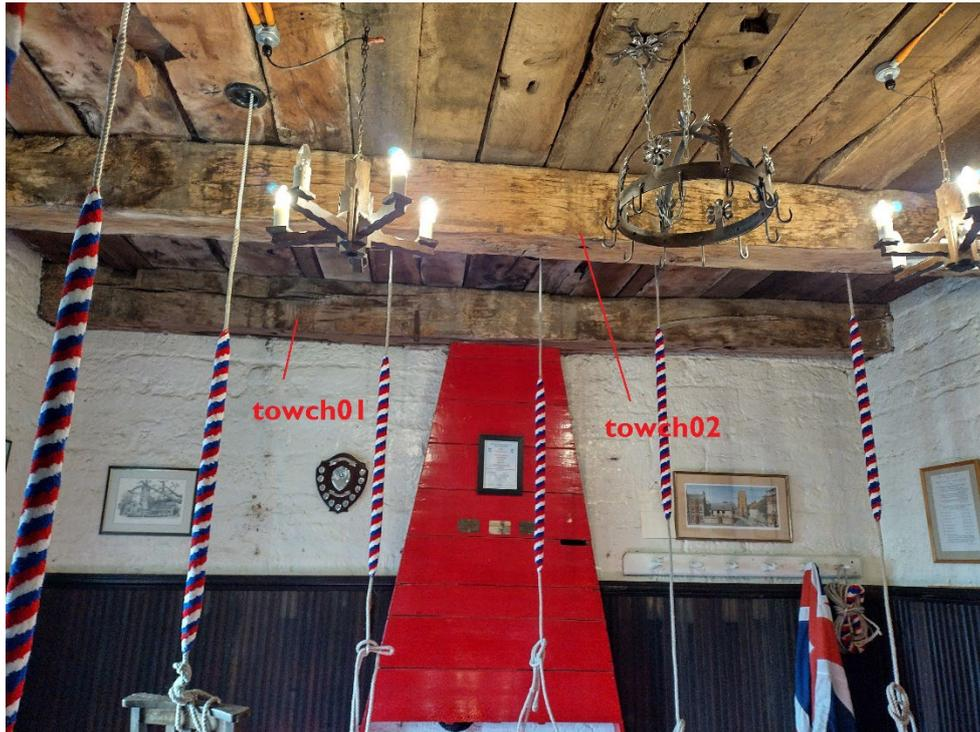
Figure 2: View of the ringing chamber ceiling, looking west, showing the timbers sampled for dendrochronology. [Photo Martin Bridge]
