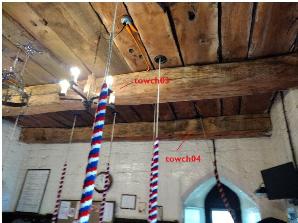
Figure 3: View of the ringing chamber ceiling, looking east, showing the timbers sampled for dendrochronology. [Photo Martin Bridge]
