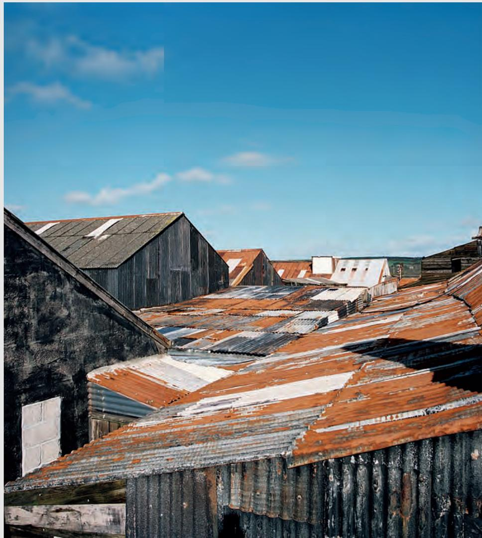
The checker-board patterns that resulted from using small sheets with uneven coatings cannot be replicated with modern corrugated-iron sheet.
