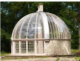
the hall and was built c 1825. Its plan is circular with a glazed hemispherical roof, with one half constructed in cast iron and the other in timber. The supporting walls are rendered masonry. The building was originally heated by an external furnace: heat was dissipated through underfloor ducts and the smoke discharged via a central stack disguised as a fluted column.
