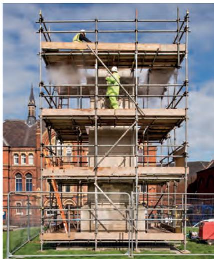
*Another form of independent scaffolding erected around Walsall Cenotaph for masonry cleaning and restoration work*
