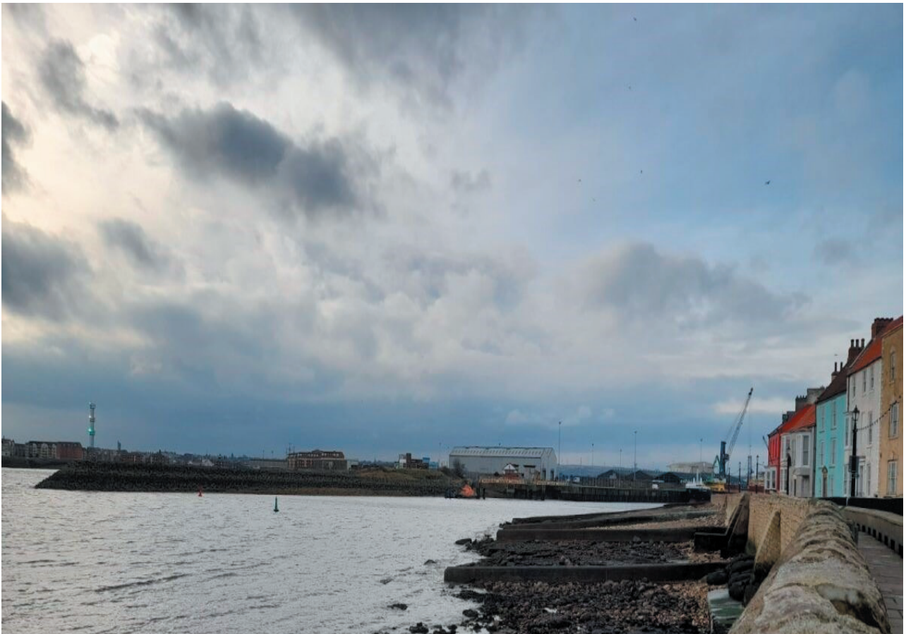
Figure 1 View from the scheduled Town Wall from the Headland © Historic England List Entry Number: 1006761
