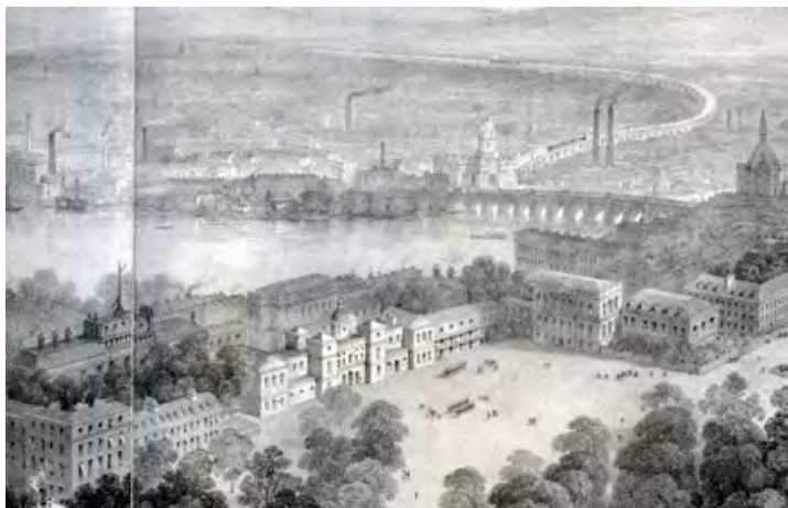
View from St James', Westminster, showing the route of the new railway, with the viaduct snaking away into the distance on the other side of the Thames.
