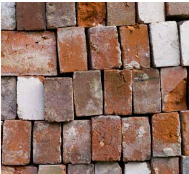
Recovered bricks at Audley End House, Essex © Historic England Ref: N080647
