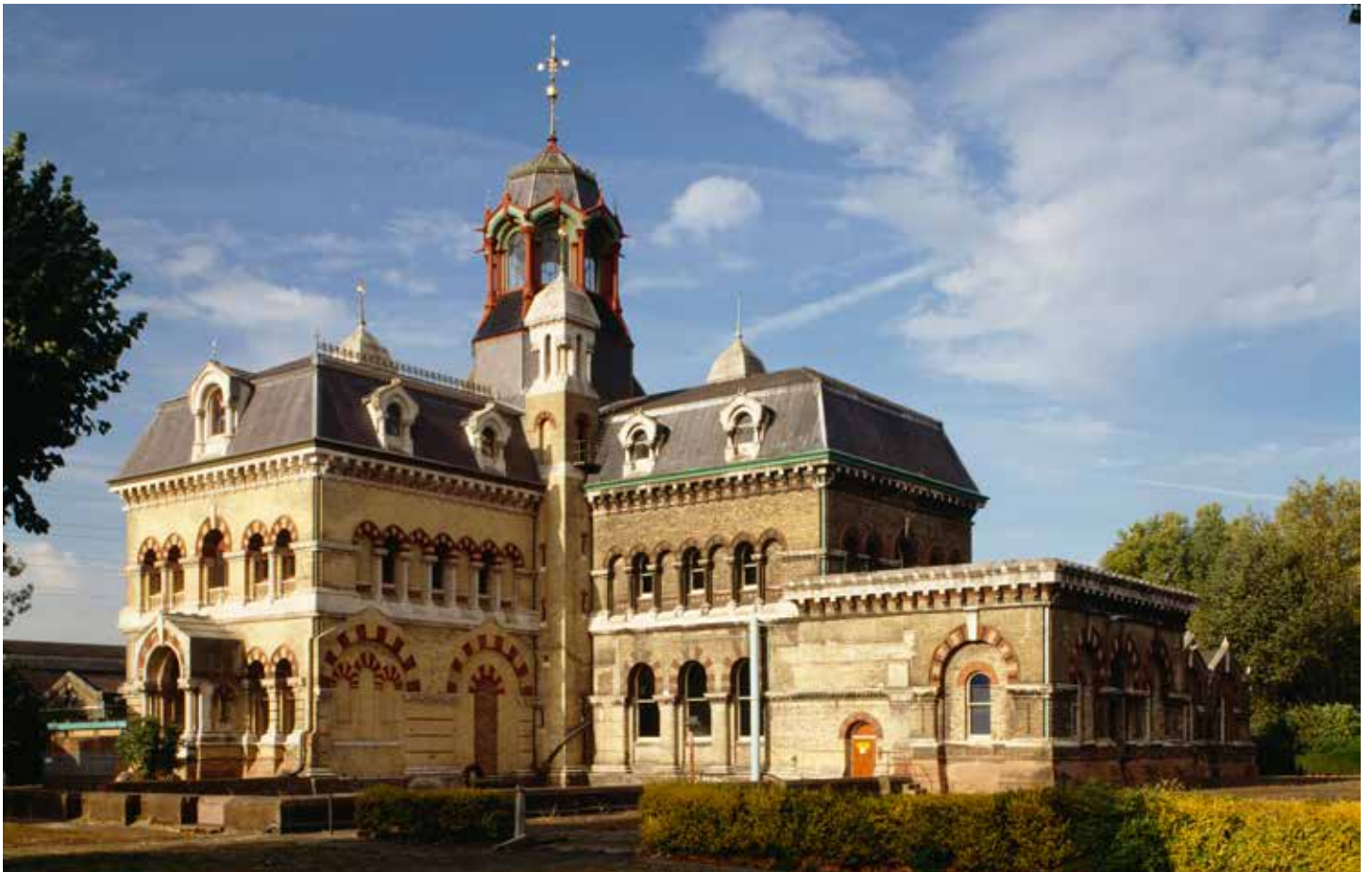
Abbey Mills Pumping Station, Newham, London © Historic England Ref: K031447
