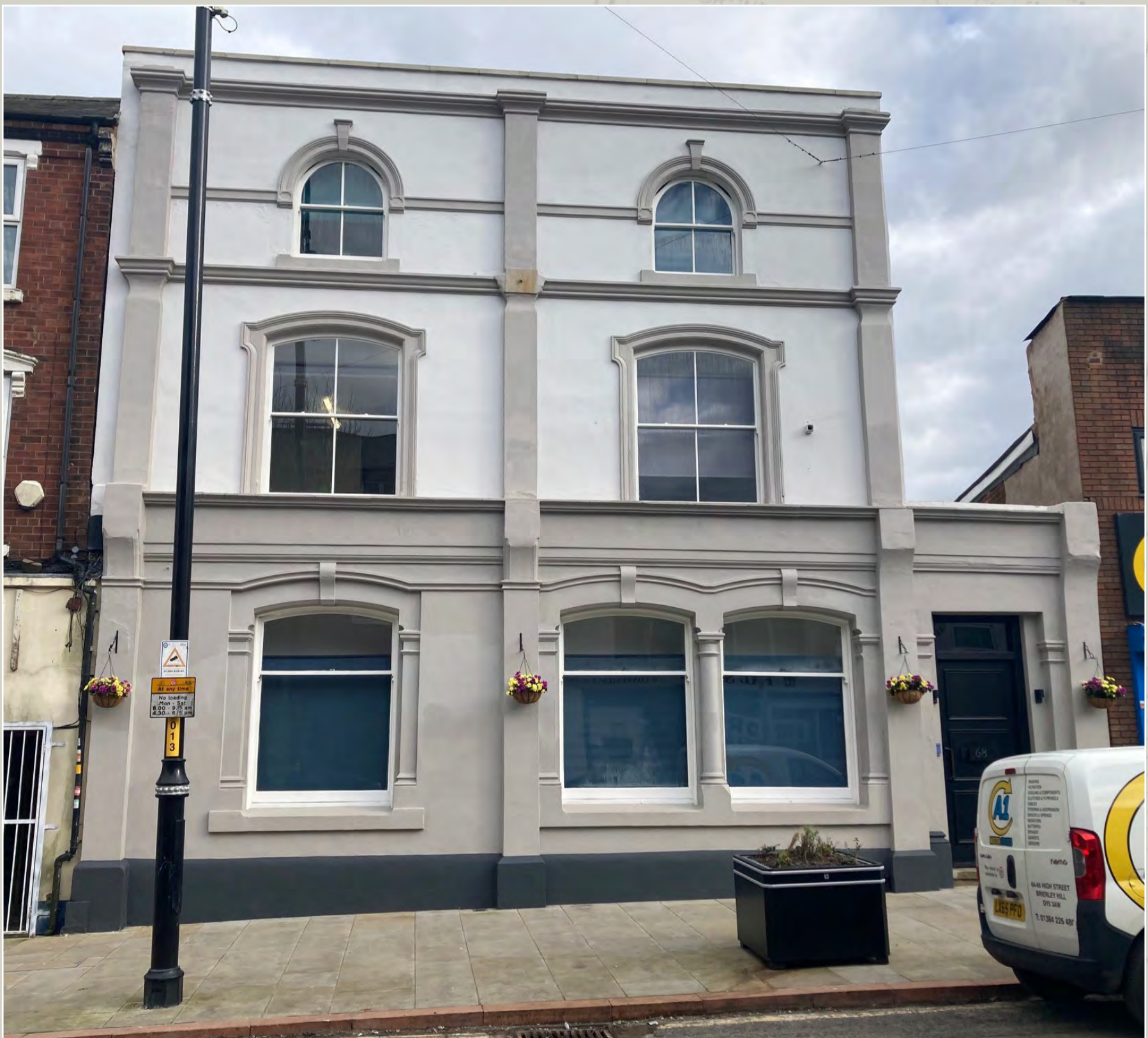
68 High Street in 2024 after it had been repaired thanks to funding through the Brierley Hill High Street Heritage Action Zone.
