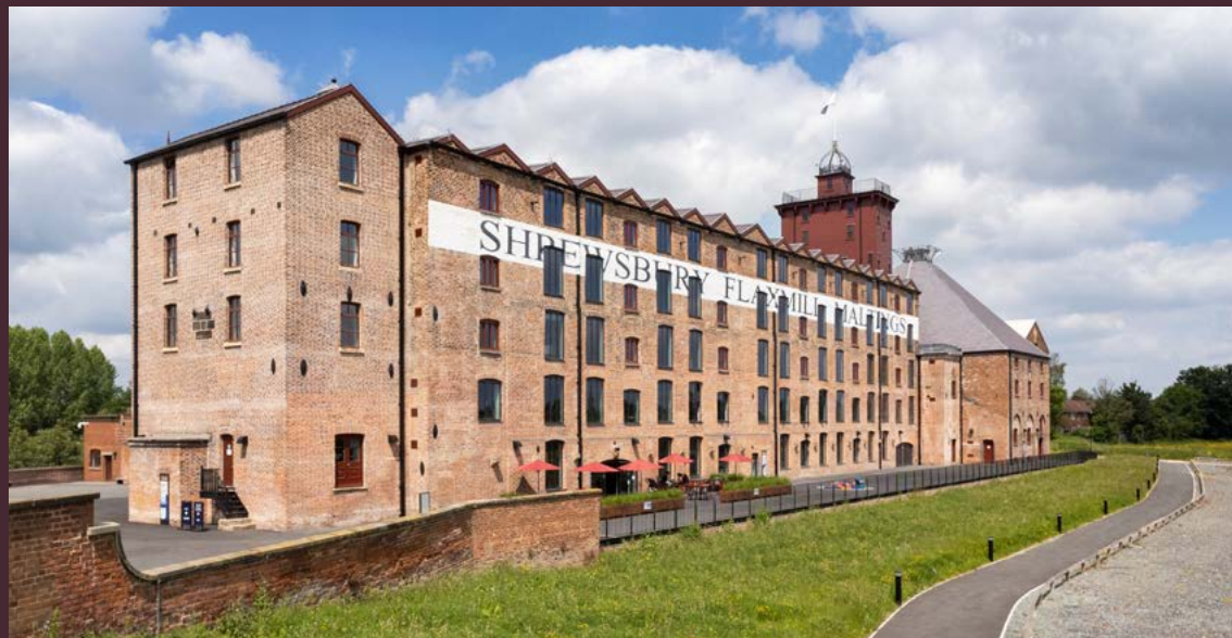
Restored Main Mill, Jubilee Tower and Kiln at Shrewsbury Flaxmill Maltings, Ditherington, Shrewsbury, Shropshire
