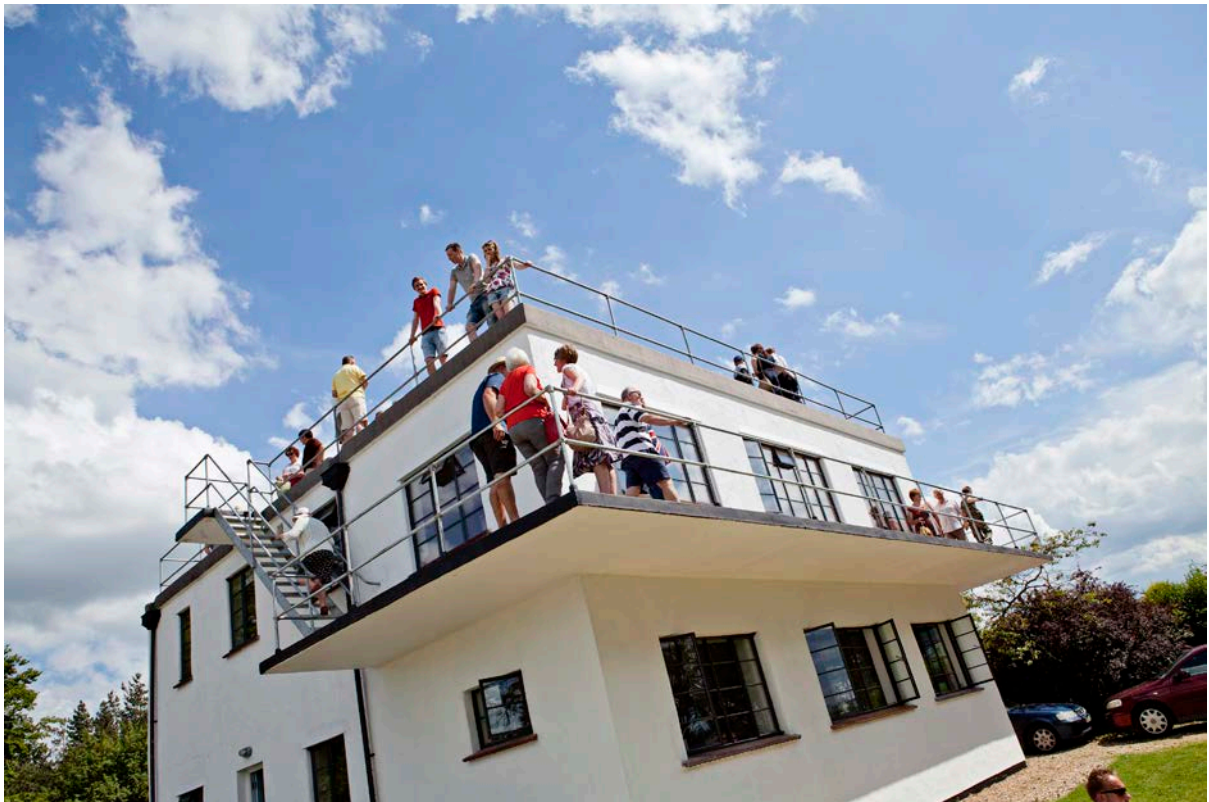
Images of the Control Tower during Heritage Open Days 2014 (photos: Paul Macro).
