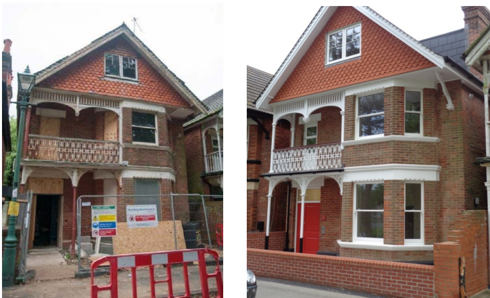
A property at Churchill Gardens – before and after. © Bournemouth Borough Council
