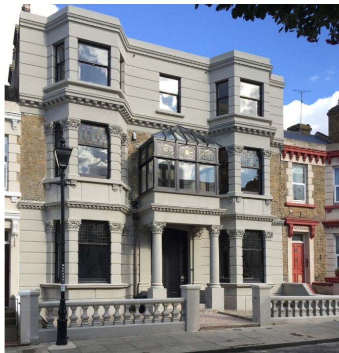
Number 12 Arthur Road, Dalby Square post renovation. © Thanet District Council
