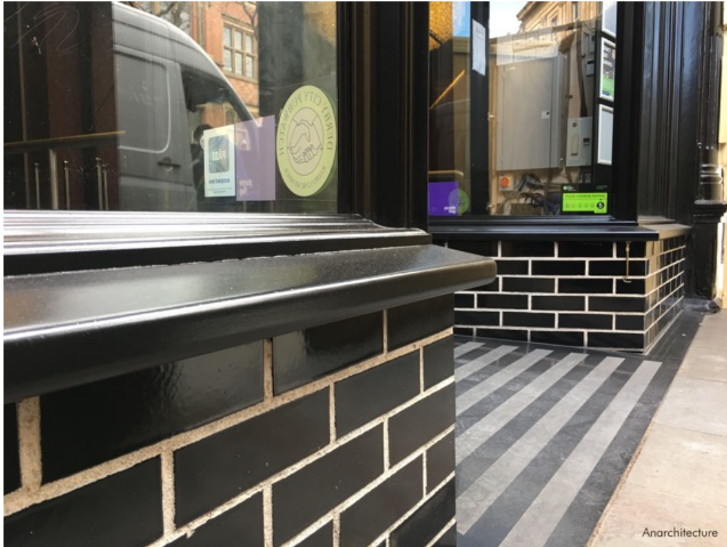
Detail of renovated shopfront on the Strand, Derby. © Anarchitecture
