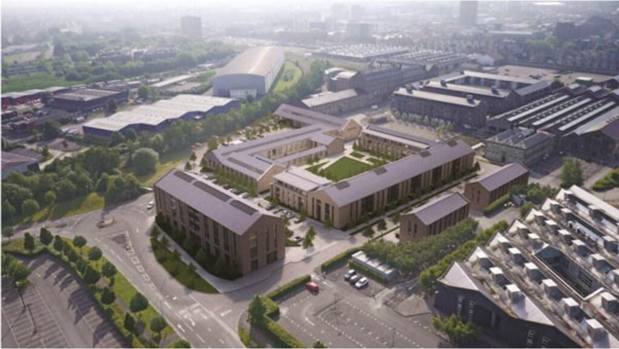
Aerial view of the former Great Western Railway Works illustrating the mix of new and original buildings. © Thomas Homes
