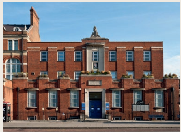
The Grade II Walworth Clinic within the Walworth Heritage Action Zone. © Historic England
