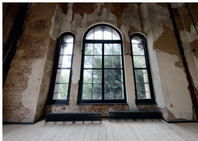
Alexandra Palace during renovation work. © Keith Armstrong
