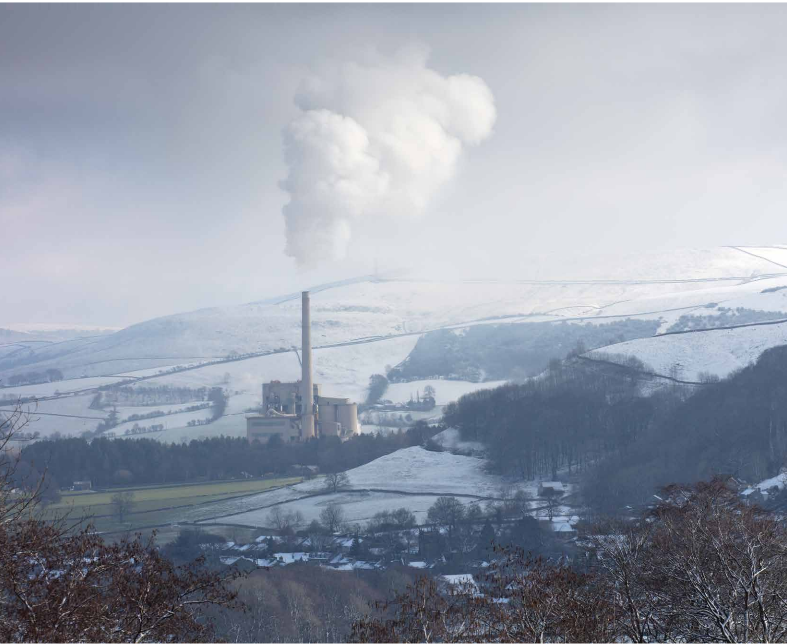
Breedon Hope Cement Works is a prominent feature in Hope Valley within the Peak District National Park. © Historic England Archive
