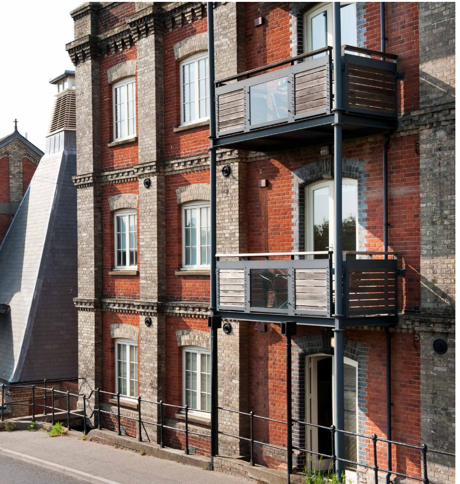
Conversion of the pre-1919 Mistley Maltings at Manningtree, Essex resulted in the preservation of significant historic buildings and the creation of new dwellings. © Historic England Archive
