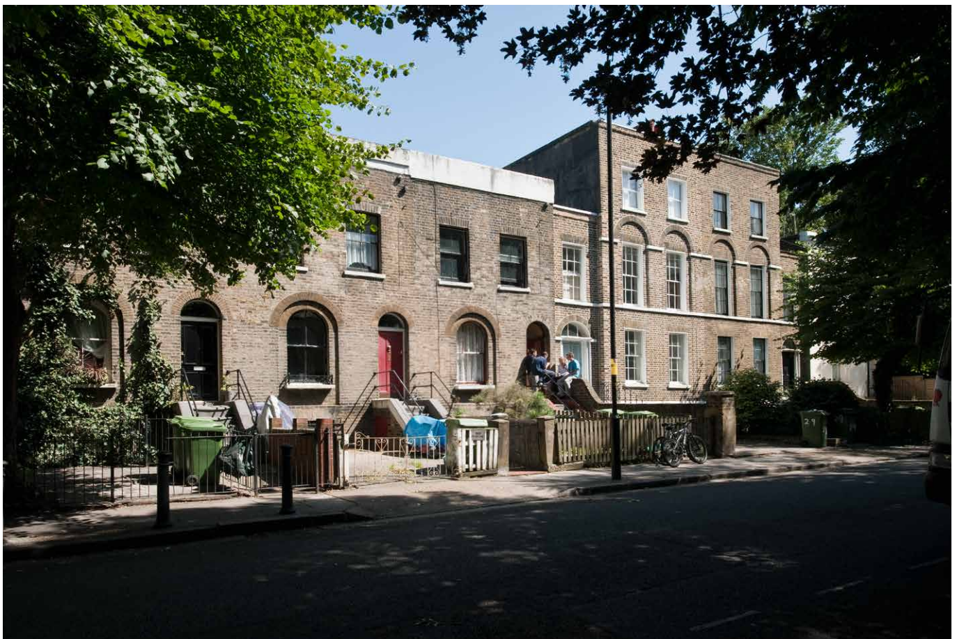
A row of terraced houses in the Old Kent Road area of Southwark, Greater London. © Historic England Archive
