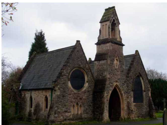
Chapel exterior before...
