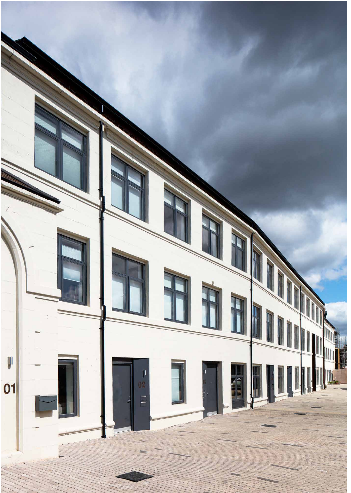
New dwellings were created at the pre-1919 Green Lane works by converting the historic industrial buildings into flats. © Historic England Archive
