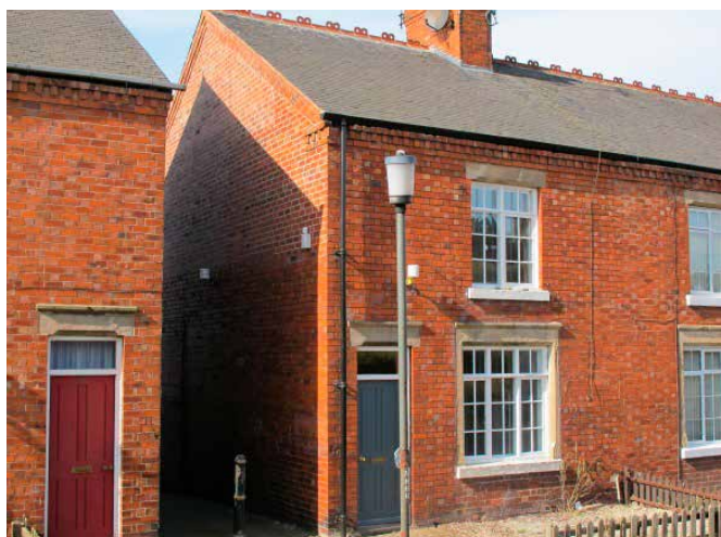
Victorian Terrace after retrofit.
