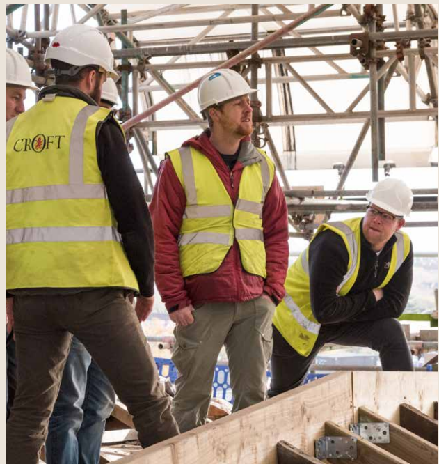
Craftspeople attending a two-day Repair and Maintenance course. © Historic England Archive
