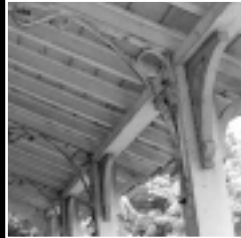
Detail of the Covered Bridge
