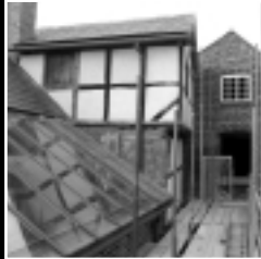
The exterior of Staircase House Stockport showing the glass roof of the viewing gallery
