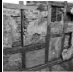
A wall at Staircase House Stockport that demonstrates construction methods
