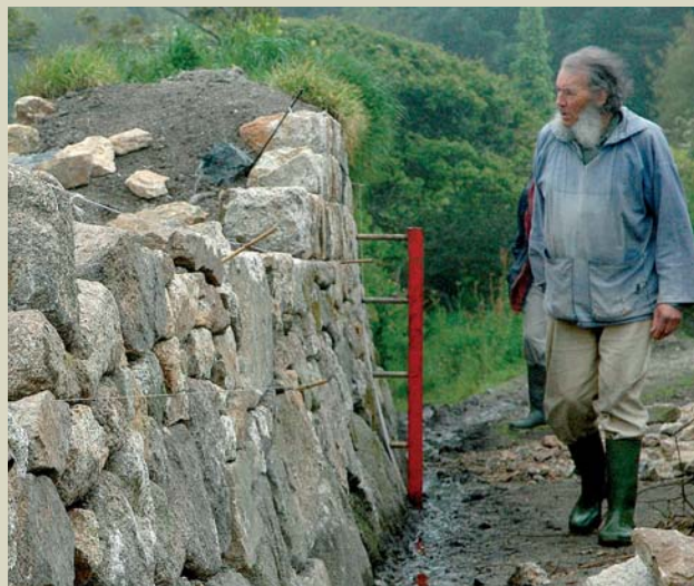
Robin Menneer, founder of the Guild of Cornish Hedgers, inspecting an apprentice-built Cornish hedge
