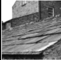
Traditional stone slate roof in the Yorkshire Dales
