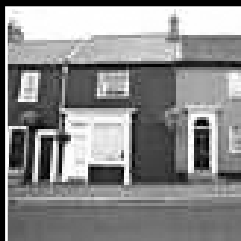
Eighteenth-century houses and shop front, Barton upon Humber conservation area
