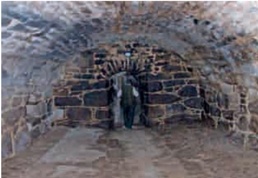
Figure 20 The stone-vaulted byre and its original byre doorway, at The Raw, near Hepple, Northumberland. [DP135347]
