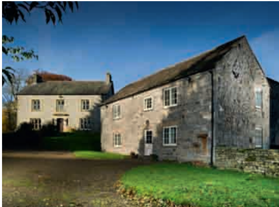
Figure 92 Low Crossgill acquired a new farmhouse in 1877 and some of the old linear farmstead was subsequently demolished, leaving a roof scar of a structure that was once thatched with heather. [DP154210]
