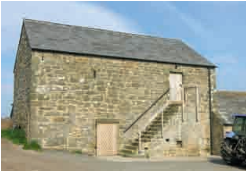
Figure 19 The much rebuilt bastle at The Raw, near Hepple, Northumberland, which eventually gained a permanent exterior stair. [DP135346]
