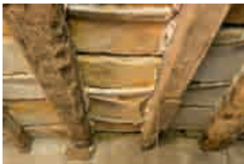
Figure 26 Large stone flags are laid on timber joists to form the floor between the byre and the living space at Annat Walls. [DP109774]
