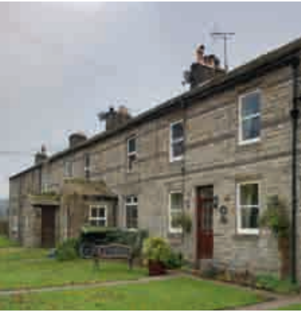
Figure 74 Cottages with banded rubble masonry on the west side of the Green, Garrigill. [DP154238]
