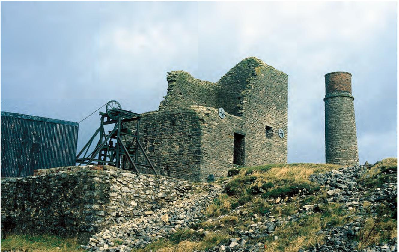
*Plate 62: Magpie Mine, Peak District, Derbyshire. Lead mining extraction occurred from the seventeenth century, until the 1960s. Most of the remains are from the later nineteenth century. The Cornish pumping engine house dates from 1868, forming part of the scheduled monument*
