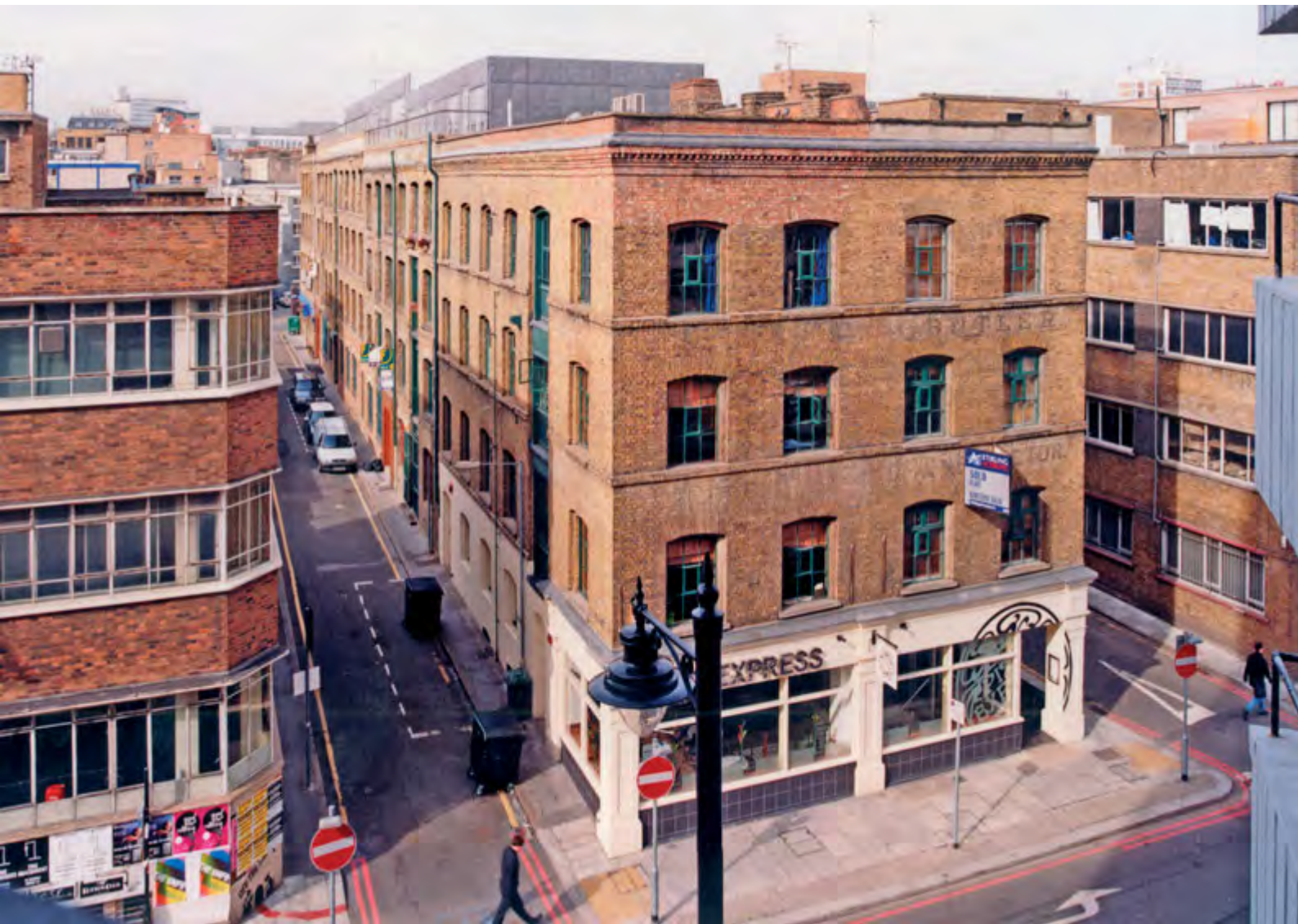
Fig 34 An island block, bounded by Christina Street, Curtain Road, Luke Street and Phipp Street, built between 1867 and 1871. The loophole bays and metal-framed windows indicate the industrial origins of the buildings but flats and restaurants now occupy what were once manufacturing spaces.
