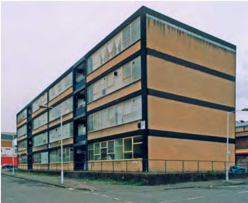
Fig 41 Part of the complex of flatted factories on Long Street, built by the London County Council in 1959. The concrete-framed blocks were provided with generously sized lifts able to take uncut sheets of plywood.
