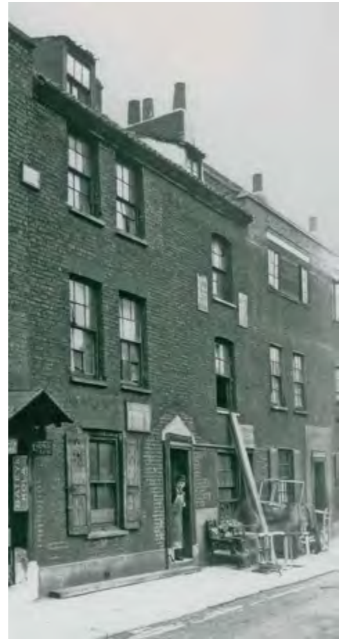
Fig 16 When 9–11 New Inn Street were photographed in 1907 all of these buildings were occupied by cabinet makers. A French polisher peers from the doorway of 9, while some chairs, finished and in skeletal form, stand on the pavement; such colonisation of the public areas for temporary storage was commonplace. (Corporation of London, London Metropolitan Archives)
