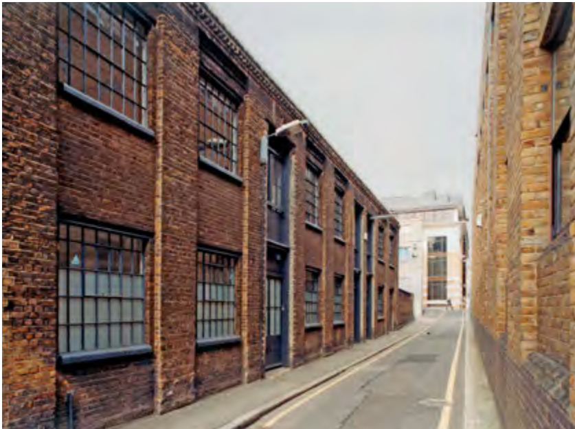
Fig 29 A group of three workshops, 8–10 New North Place, dating from 1895. The interiors are restricted in size as the buildings are quite shallow in depth, suitable only for small-scale businesses.
