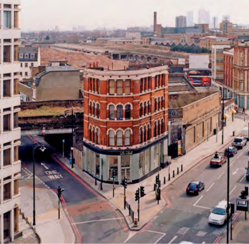
Fig 8 10 Great Eastern Street was built in 1879. Its wedge-shaped site was the result of having cut the new road across an existing street pattern. Behind passes the disused viaduct of the North London Line while beyond lies the remains of the Bishopsgate Goods Station.
