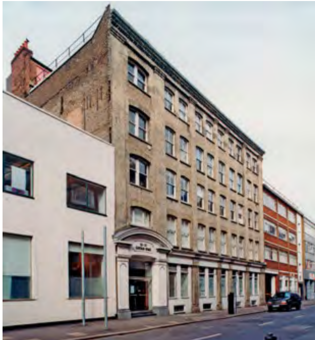
Fig 21 13–19 Curtain Road, built in 1861 for J B Richards, is one of the earliest examples of a fully developed showroom-warehouse. In 1881 the building became the showrooms and offices of B Cohen and Sons, one of the leading wholesale manufacturers and exporters in the district.
