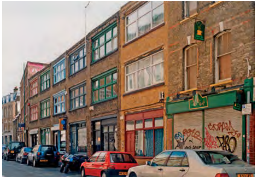
Fig 38 An industrial terrace of six workshops, 16–26 Rivington Street, built in 1897. Utilitarian in appearance, they were apparently constructed with flat roofs possibly to allow for additional storeys.
