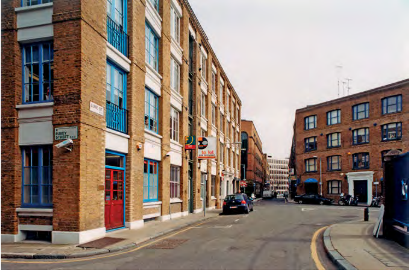
Fig 4 Former workshops of the 1870s and 1880s on Luke Street and Phipp Street, built primarily for the furniture trade. Close to the main thoroughfares, these manufacturing spaces were used by many kinds of businesses including small-scale manufacturers and wholesalers with showrooms nearby.
