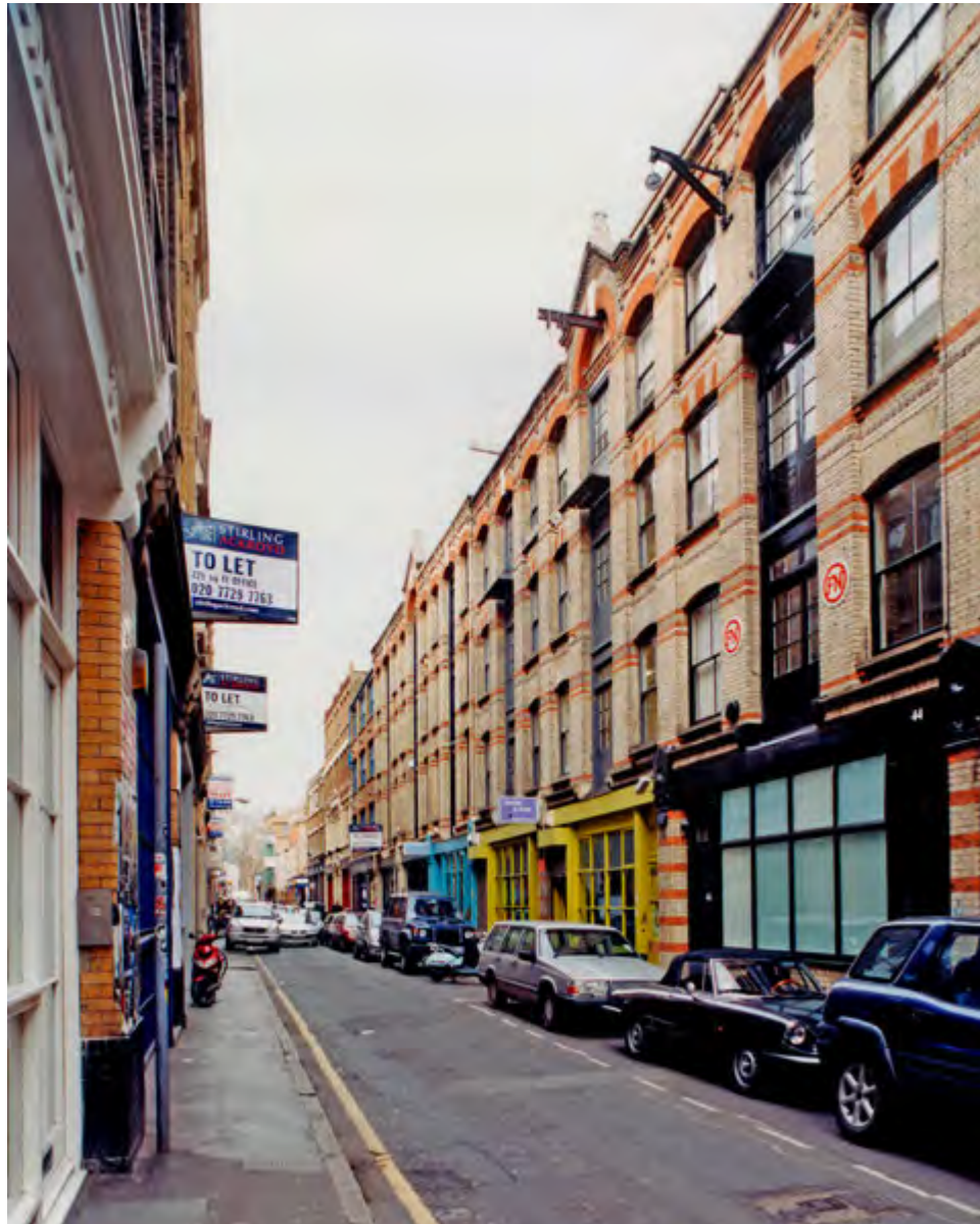
Fig 36 One of the most impressive workshop developments in the area, 43–49 Charlotte Street, was developed between 1877 and 1881. Furniture making and furnishing continued in these buildings until at least the 1950s.
