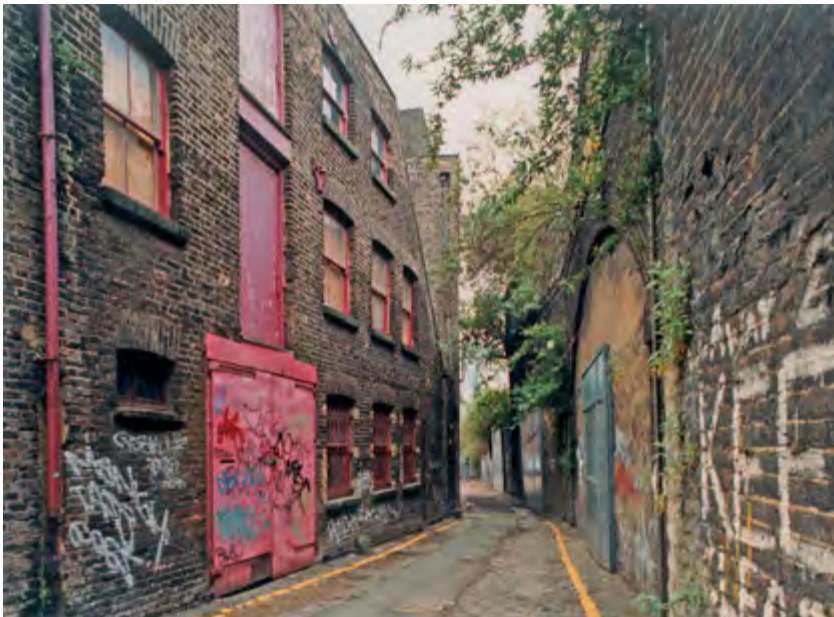
Fig 37 A back-alley workshop, probably dating from the 1870s, in Bowl Court off Shoreditch High Street. The arches of the adjoining railway viaduct were also used as workshops and timber stores.
