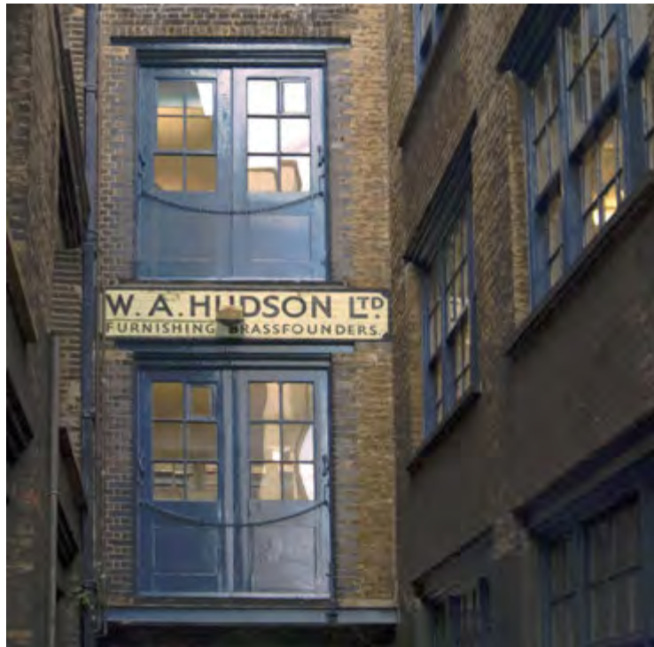
Fig 50 Loading doors at the rear of 55 Charlotte Road, the painted signage of the building's former occupant still prominent. Until the 1980s W A Hudson continued to occupy a site spread over many properties, the full extent of which can be seen in Fig 10.
