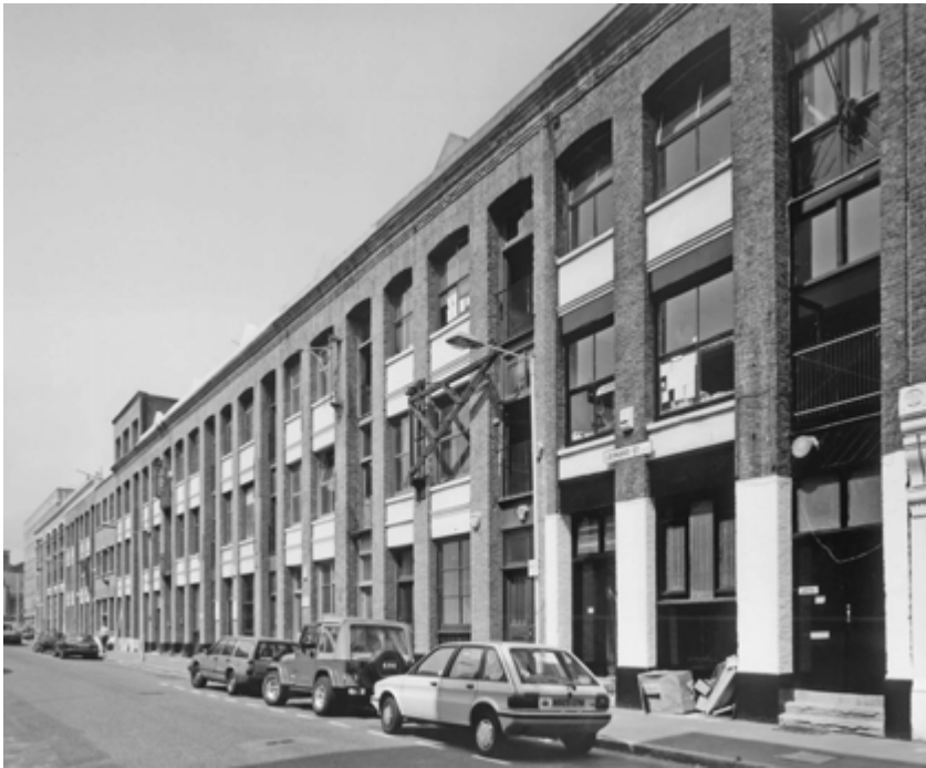
Fig 35 The impressive terrace of workshops, 65–83 Leonard Street was built between 1874 and 1877. Its impact derives partly from the great length of unified façade and the powerful rhythm of its closely spaced arcade of brick piers. Each property has a three-bay frontage, with windows flanking a loophole bay. The group retains a variety of iron or steel wall cranes of various dates.
