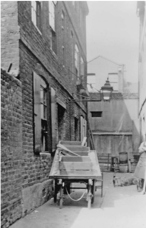
Fig 30 This alley off Cheshire Street in Bethnal Green, 3–9 Hare Court, was built as weaver's housing around 1725. The presence of a barrow containing part-assembled drawers indicates that in 1928, when the photograph was taken, at least one of the residents was a cabinet maker. (© Crown copyright.NMR)
