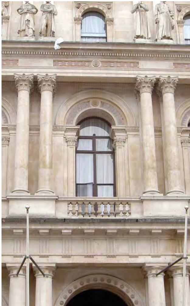
South elevation of quadrangle showing brown staining on columns
