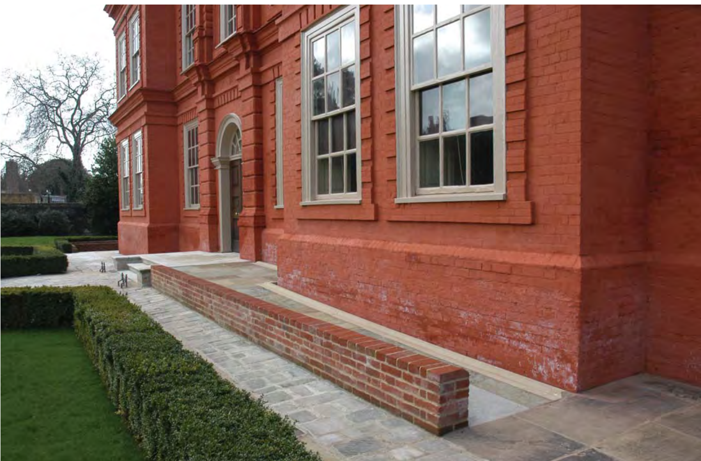
The new access slope outside the front entrance to Kew Palace. The slope is hidden from long views of the palace by the formal box hedging.
