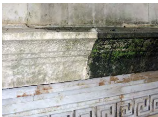
Results of DOFF cleaning on the south elevation of the quadrangle, before (right) and after (left)
