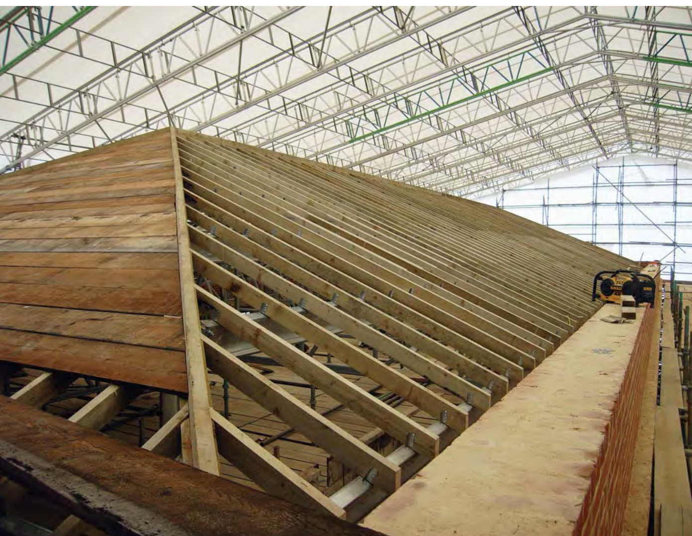
Work in progress on the new roof and brick parapets of the north wing of the Block Mills
