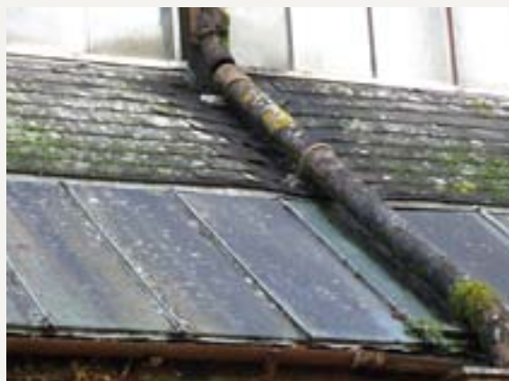
RAF Bicester: One of the hangars, showing the failing roof
