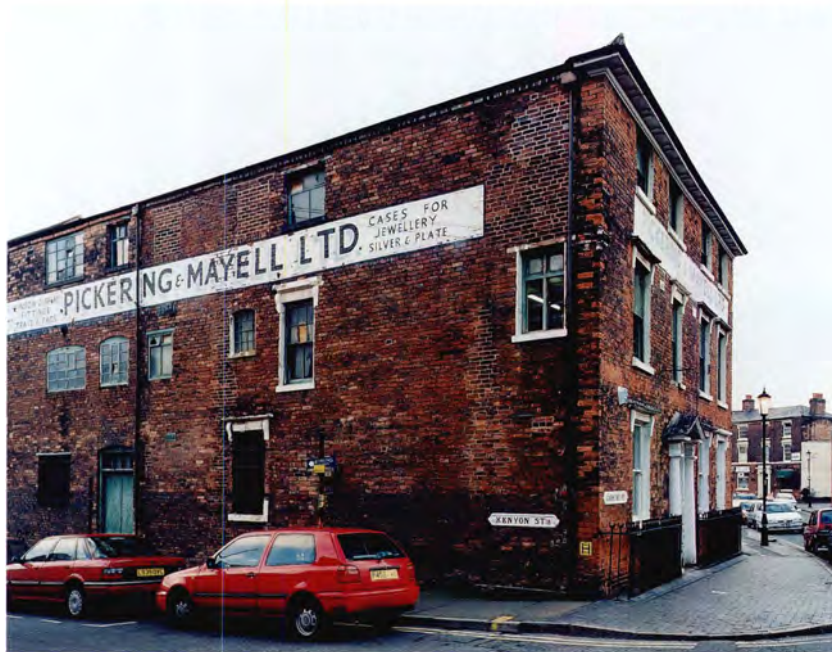
Fig 6 (left) The Reliance Works of Pickering & Mayell Ltd at No. 42 Caroline Street was built as a pair of houses with rear workshops in around 1826. The workshops of No. 42, which retain some of their original wooden-framed multi-pane windows, face onto Kenyon Street. [AA98/18072]
