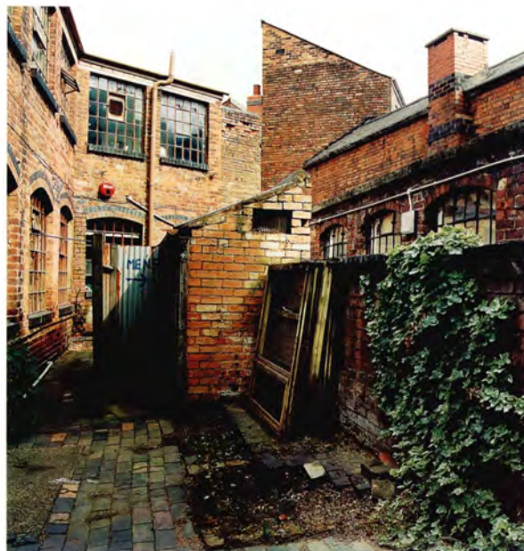
Fig 9 (above left) Walker Pressings, No. 89 Vyse Street, a converted terraced house of about 1850. A workshop with extensive glazing has been created in the former attic of the house. [AA99/08835]
