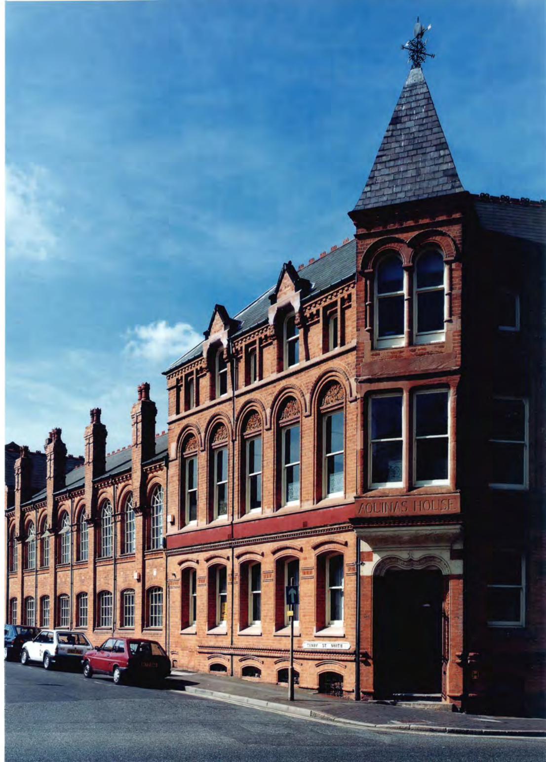
Fig 11 The Italianate-style former jewellery factory of Manton and Mole, now Aquinas House, built in 1882 on the corner of Warstone Lane and Tenby Street North. This state of the art works consisted of a three-storey corner block (right) containing offices and warehouses, and an adjoining two-storey workshop range (left). The latter fronts onto the street and was therefore treated architecturally. The building has recently been converted to a variety of uses including jewellery workshops and an architects' office. [BB99/04721]
