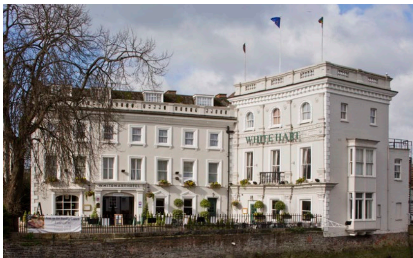
Figure 78 The White Hart became the premier hotel in the town and was extended to take over the building seen on the right, which was recased c 1878 in an elaborate confection of moulded stucco, disguising the plain Georgian structure underneath. [DP161446]
