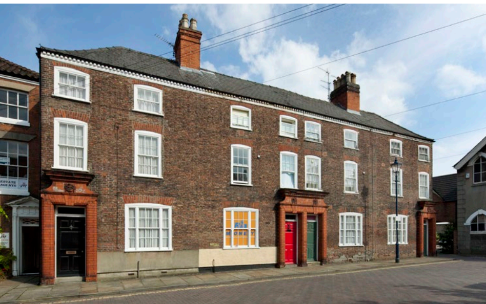
Figure 32 (left) Nos 7–10 Pump Square with dentilled eaves and almost flush sash windows of the mid-18th century. The late 19th-century door surrounds add an incongruous note. [DP161468]
