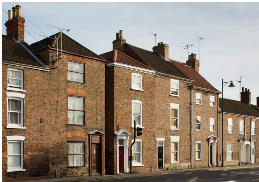
Figure 45 Nos 38–44A Pen Street. Typical of much late 18th and early 19th-century development in the area, these were tall narrow houses, mostly built by individual speculators, as may be seen by the breaks in the brickwork between each house. No 44A is a reconstruction. [DP165423]
