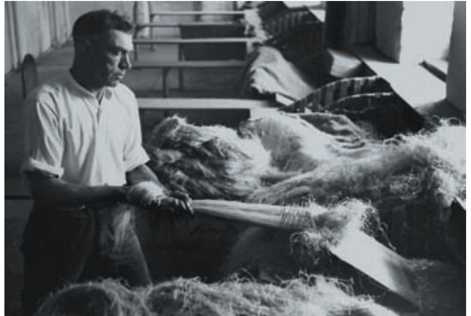
Figure 10 Drawing hemp by hand in a Bridport Mill. [Museum of Net Manufacture]
