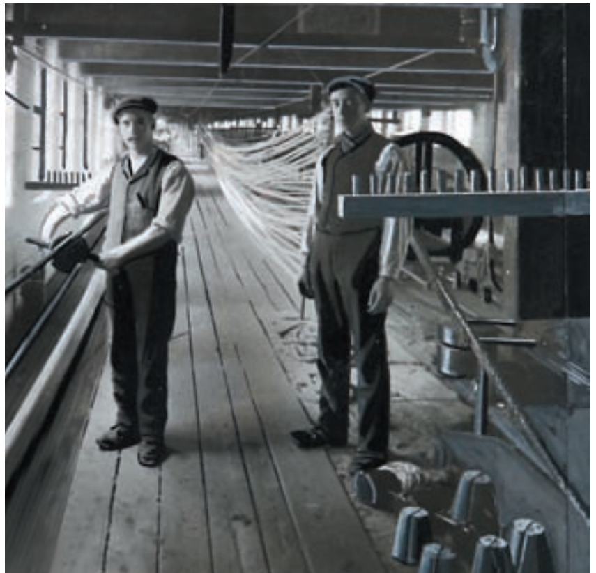
Figure 20 A rare 19th-century photograph (hand tinted) showing the interior of a Bridport covered walk. [Museum of Net Manufacture]
