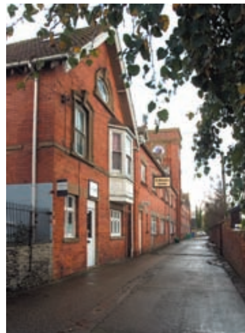
Figure 41 The alley behind No. 40 St Michael's Lane was formerly an open walk. The two-storeyed late 19th-century building on the left is now the best-preserved covered walk in the central part of Bridport; similar buildings on the right were replaced by north-light sheds in the 1920s. [DP001484]
