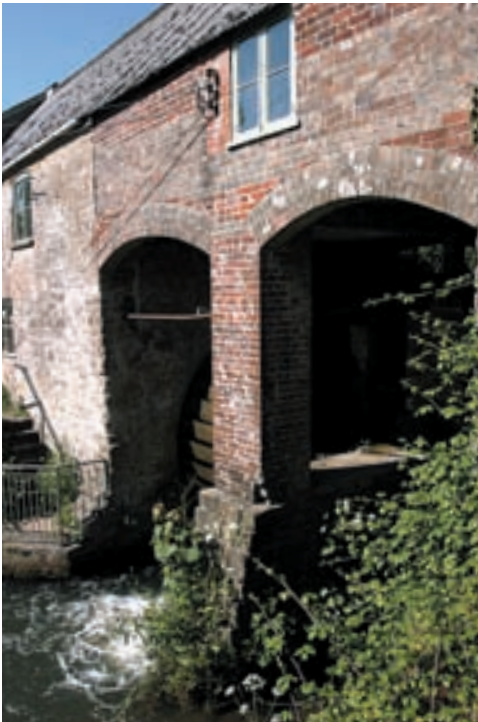
Figure 52 The wheel chamber of Mangerton Mill supplied power for both the mill stones and the flax-processing machinery, which were located in separate rooms on either side of the race. [DP005175]
