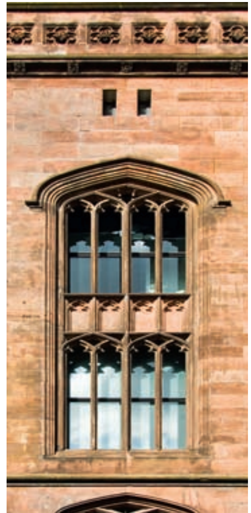
Figure 90 The Collegiate Institution, Shaw Street: modern glazing has been recessed behind the original mullions and transoms. [DP039412]
