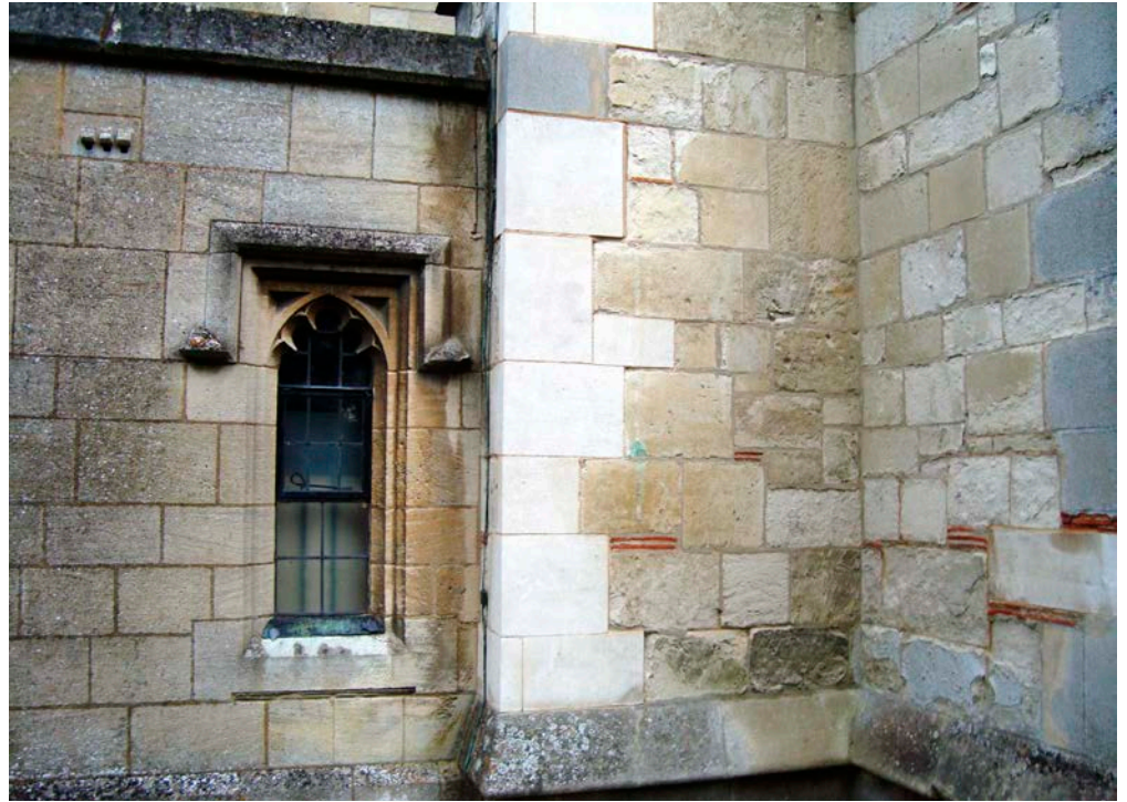
Figure 15: Church of St Mary, Eaton Bray. Totternhoe Stone ashlar blocks.
