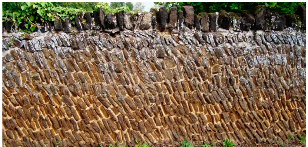
Figure 9: Boundary wall at Village Farm, Sutton. Lower Greensand stone.
