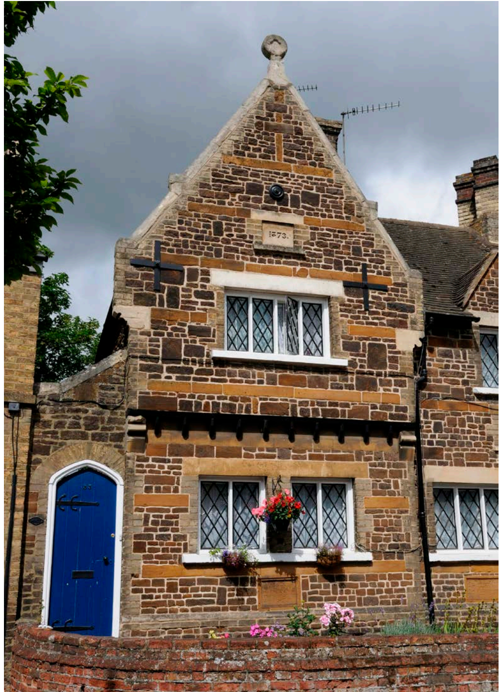
Figure 13: Wilkes Almshouses, Leighton Buzzard. Lower Greensand stone.
