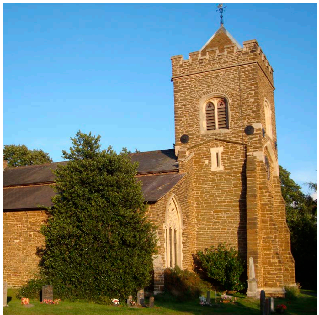
Figure 11: St Mary's Church, Maulden. Lower Greensand stone.
