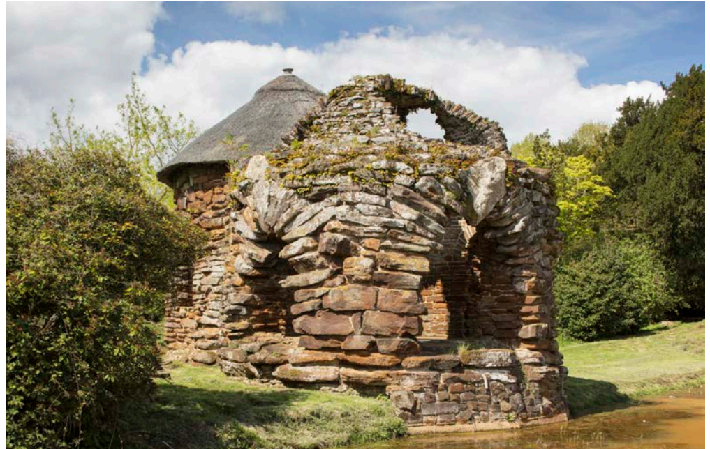
Figure 2: Wrest Park bath house, Silsoe. Local carstone.
