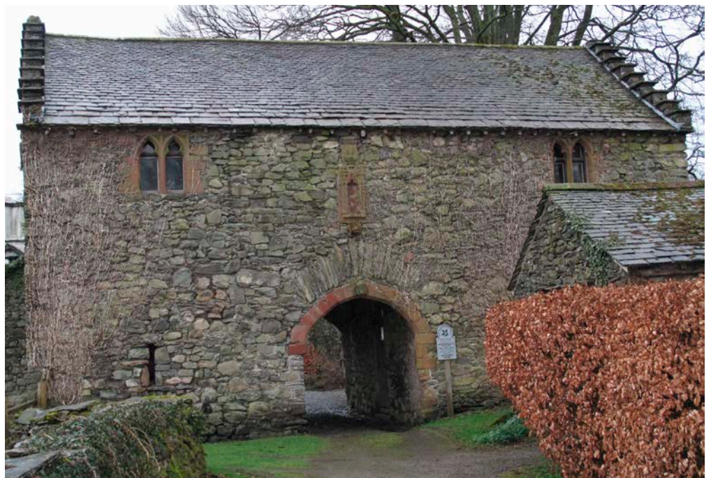
Figure 21: Hawkshead Old Courthouse, Ambleside. Borrowdale Volcanic Group rubblestone and boulders and Permo- Triassic sandstone.
