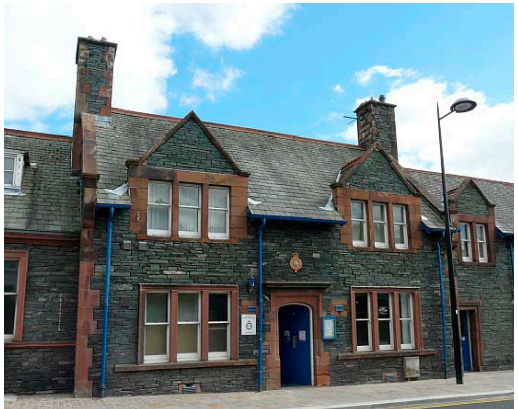
Figure 3: Former police station and adjoining Magistrates Court, Keswick. Borrowdale Volcanic Group slate and Permo-Triassic sandstone.
