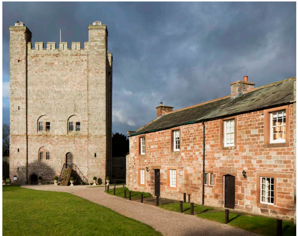
Figure 11: Terraced cottages, Appleby-in-Westmorland. Yoredale Group and Permo-Triassic sandstones. Caesar's Tower. Local Carboniferous sandstone.
