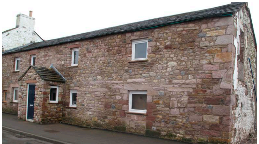
Figure 18: Dwelling in Brough. Fieldstones and/or stream boulders.
