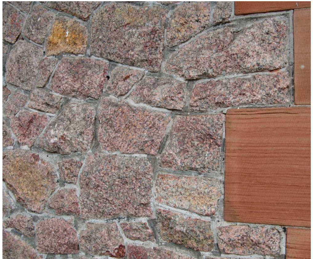
Figure 6: Railway station, Millom. Eskdale Granite blocks with dressings and bands of red-brown Sherwood Sandstone.
