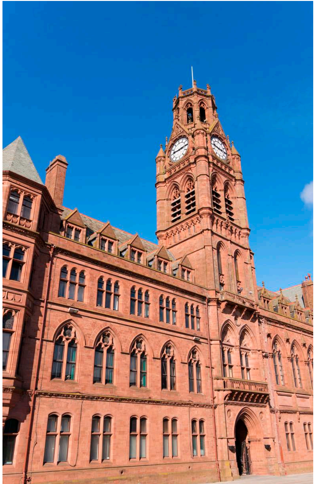
Figure 16: Furness Town Hall, Barrow-in-Furness. Sherwood Sandstone.
