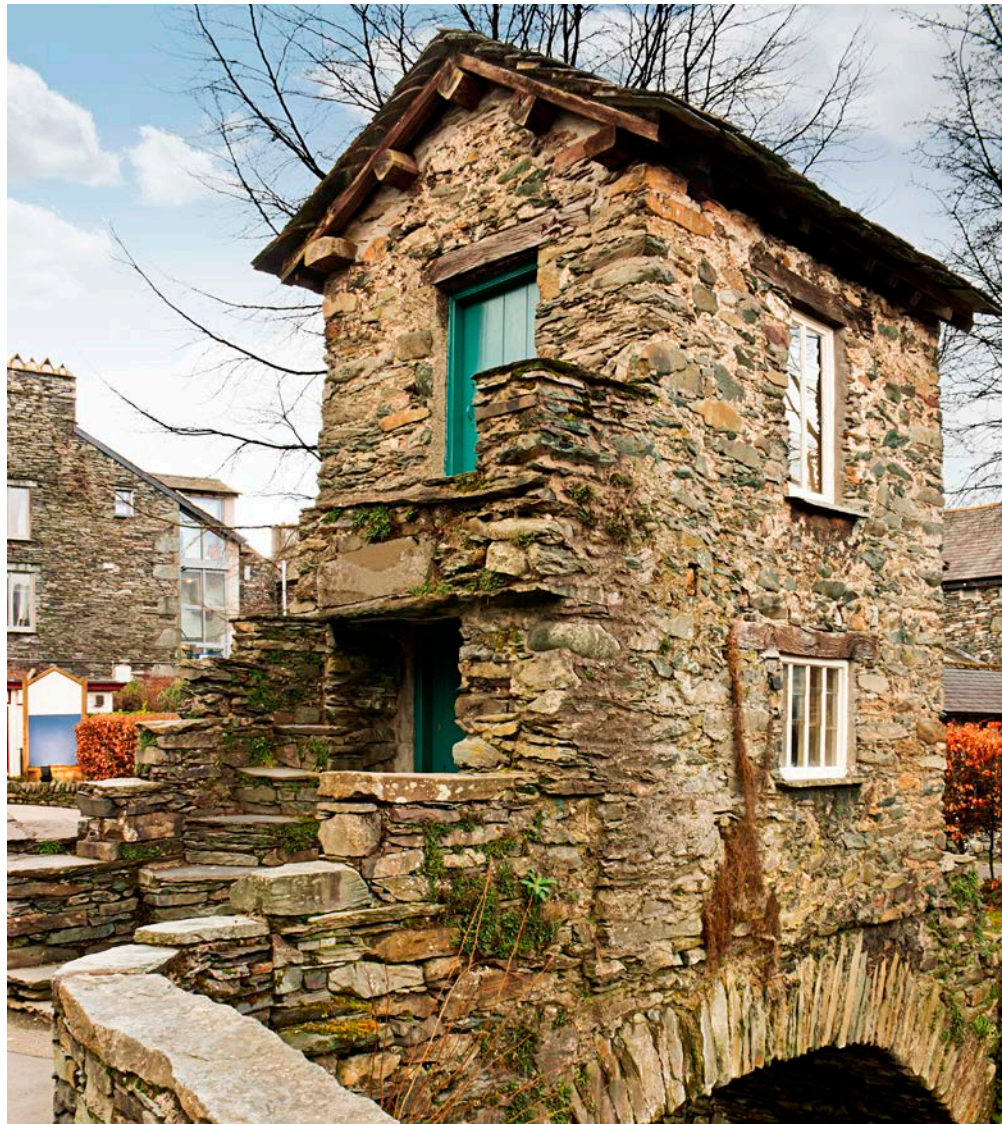
Figure 4: Bridge House, Ambleside. Borrowdale Volcanic Group rubblestone, including vesicular andesite.
