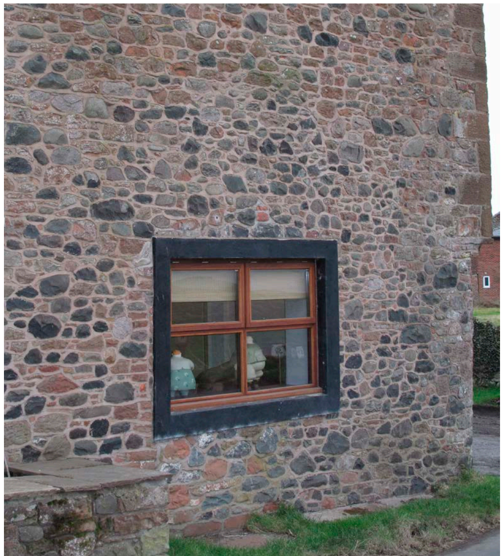
Figure 19: Cottage, Port Carlisle. Rounded boulders and cobbles.
