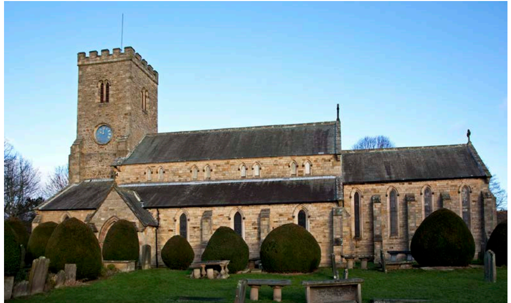
Figure 5: Church of St Mary and St Stephen, Wolsingham. Stainmore Formation Sandstone.
