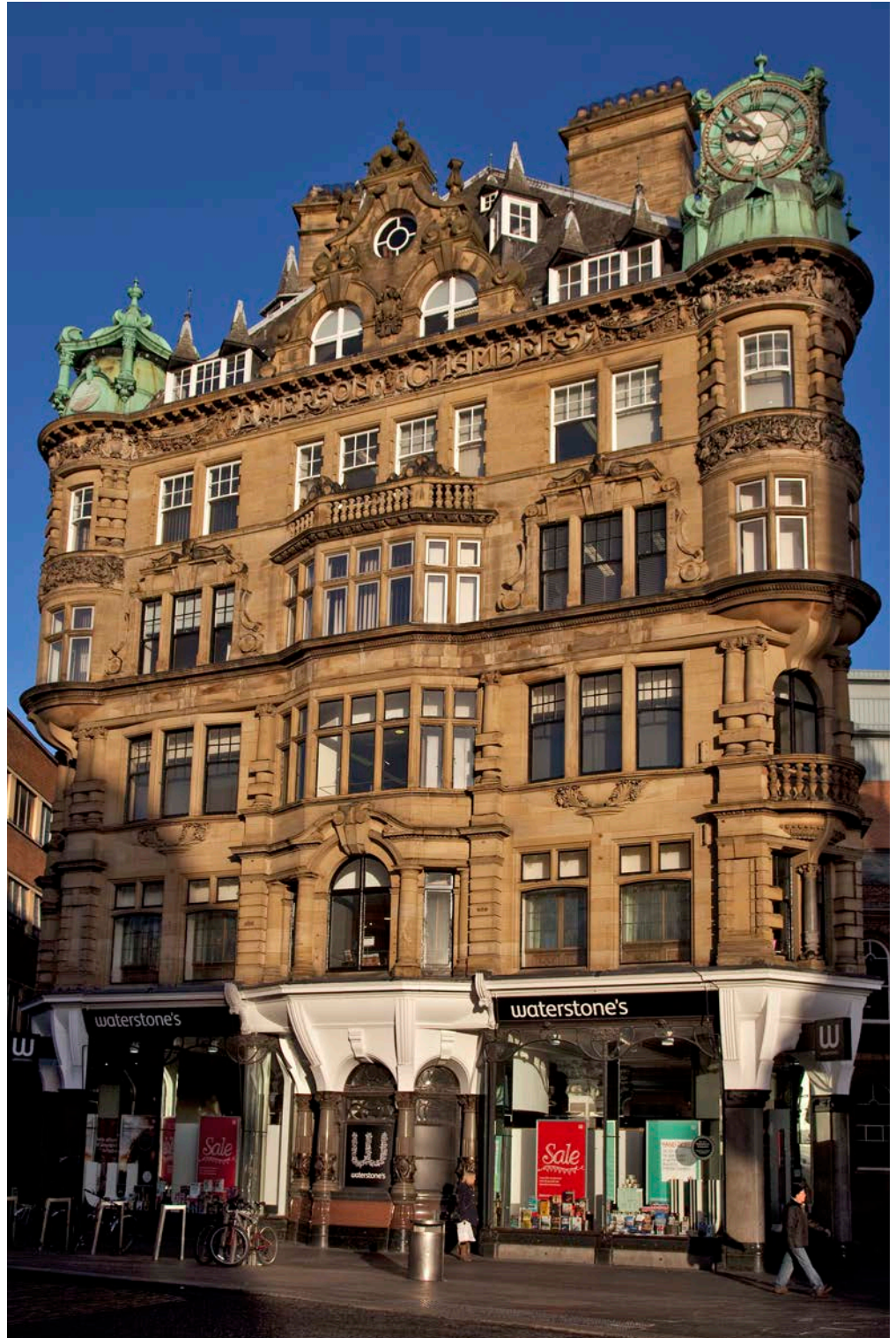
Figure 12: Emerson Chambers, Blackett Street, Newcastle upon Tyne. Middle Coal Measures Sandstone.
