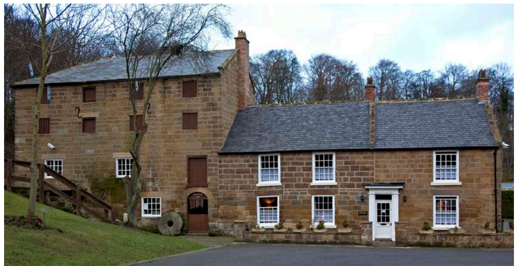
Figure 18: Tocketts Mill and Mill House, Guisborough. Saltwick and Cloughton Formations Sandstone.
