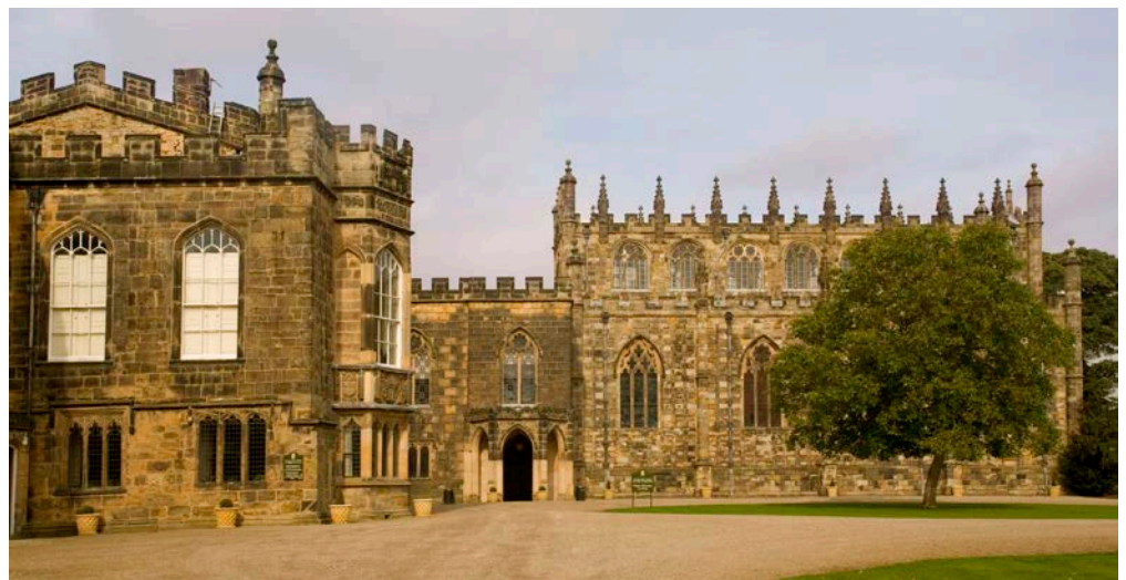
Figure 11: St Peter's Chapel, Auckland Castle, Bishop Auckland. Pennine Middle Coal Measures Formation Sandstone.
