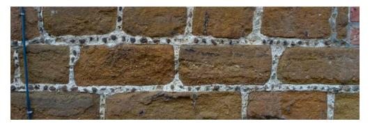
Figure 17: Carstone with galletted mortar joints
