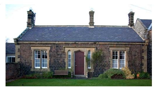
Figure 28: Dolerite coursed masonry.
