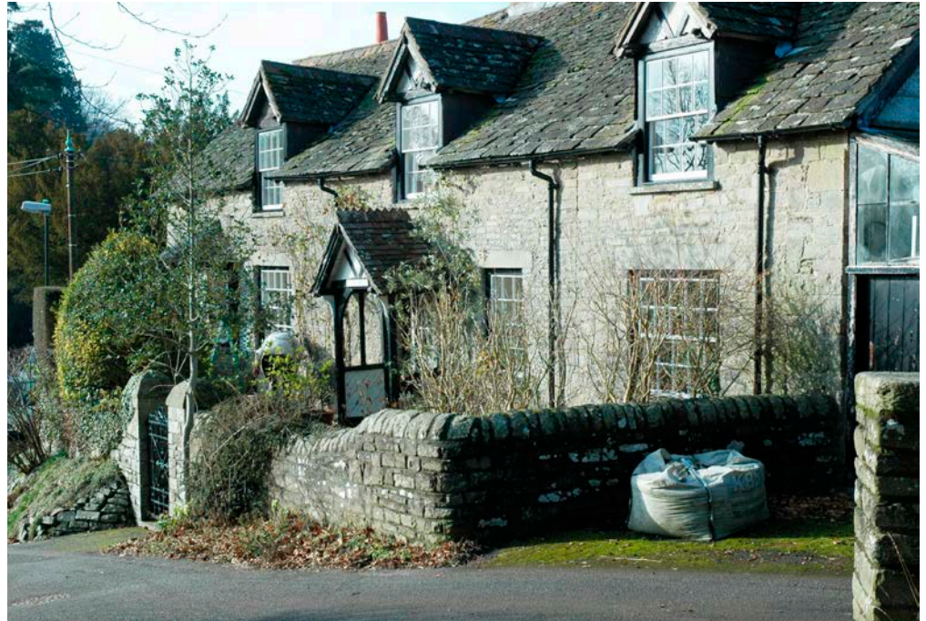
Figure 22: Flagstone roofs. Raglan Mudstone Formation.
