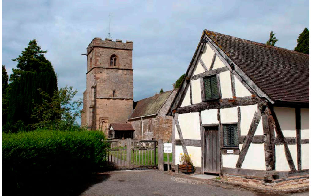
Figure 1: Timber framed building, Colwall. Stone sole plate.
