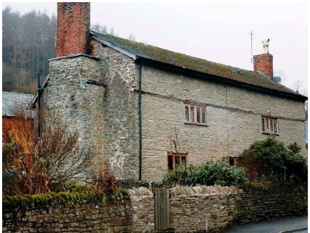
Figure 13: Farmhouse and boundary walls. Aymestry Limestone.
