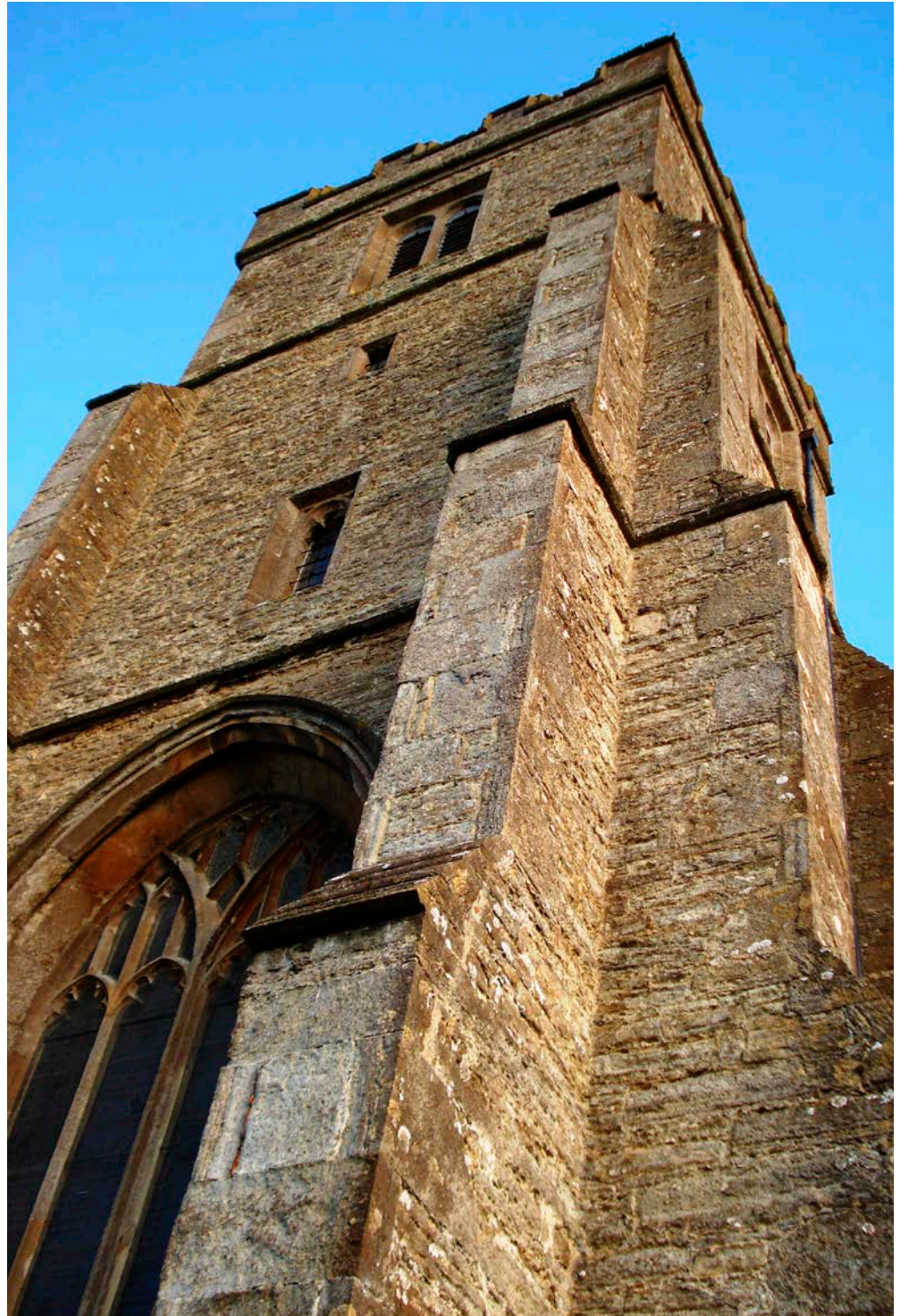
Figure 9: All Saints Church tower, Biddenden. Bethersden Marble.
