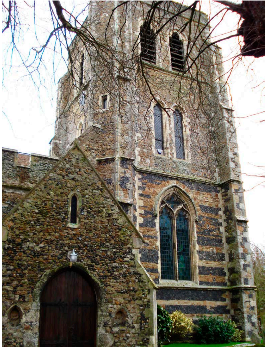
Figure 23: Church of St Martin, Herne. Septaria nodules, knapped flint and Thanet Sandstone.
