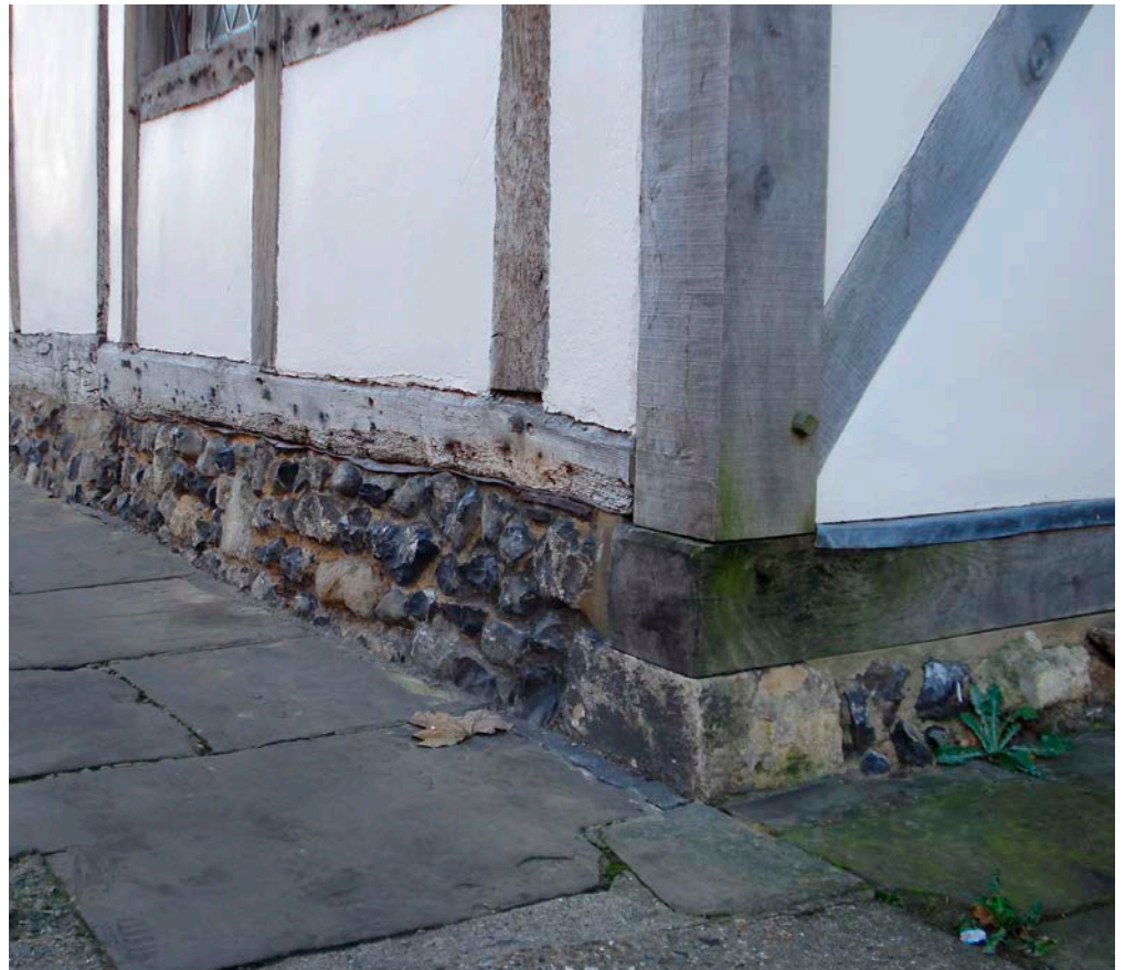
Figure 17: Timber frame building, Canterbury. Flint plinths.
