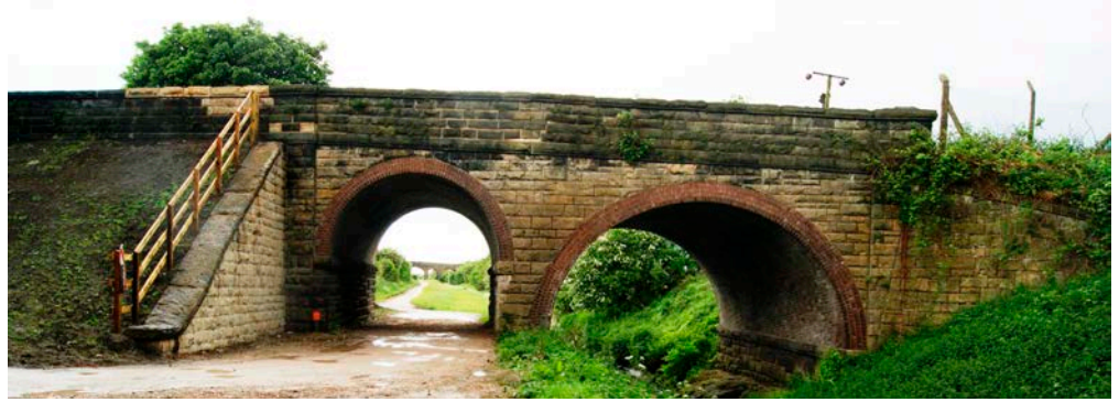
Figure 28: Great Altcar railway bridge. Ormskirk Sandstone.
