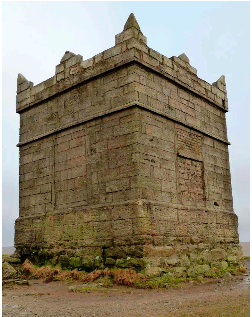
Figure 20: Tower, Rivington Pike. Rough Rock.
