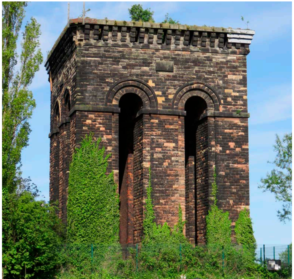
Figure 30: Water Tower, Tower Hill, Ormskirk. Ormskirk Sandstone.
