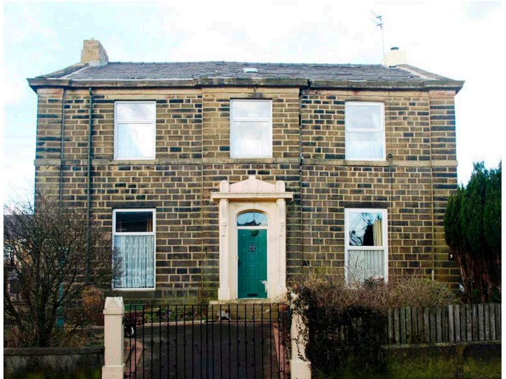
Figure 23: House, Clayton-le-Moors. Old Lawrence Rock.
