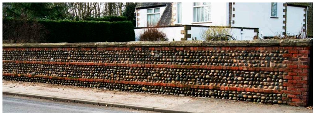
Figure 31: Lytham Hall boundary walls. Cobbles.
