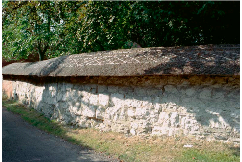
Figure 13: Boundary wall. Chalk clunch with a tile capping and flint base.
