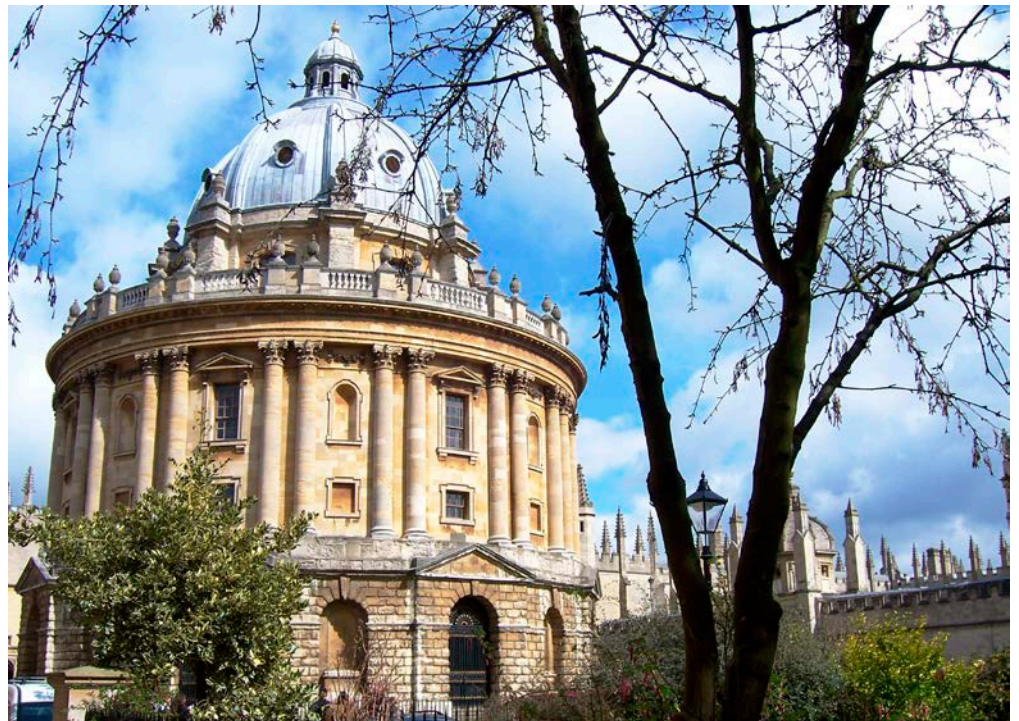
Figure 7: Radcliffe Camera, Oxford. Headington Freestone used on lower storey.
