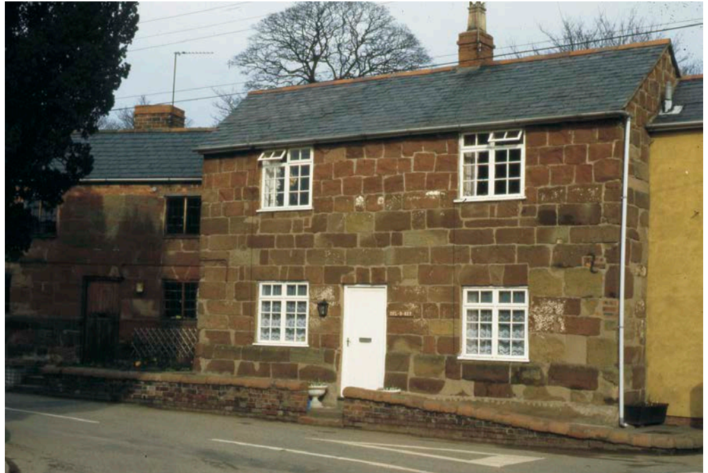
Figure 49: Cottage, Myddle. Wilmslow Sandstone.
