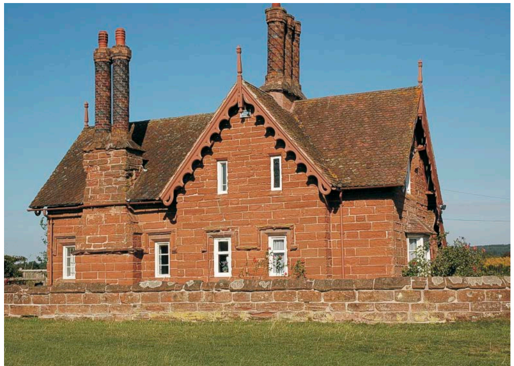
Figure 48: Dudmaston Gate Lodge. Bridgnorth Sandstone.
