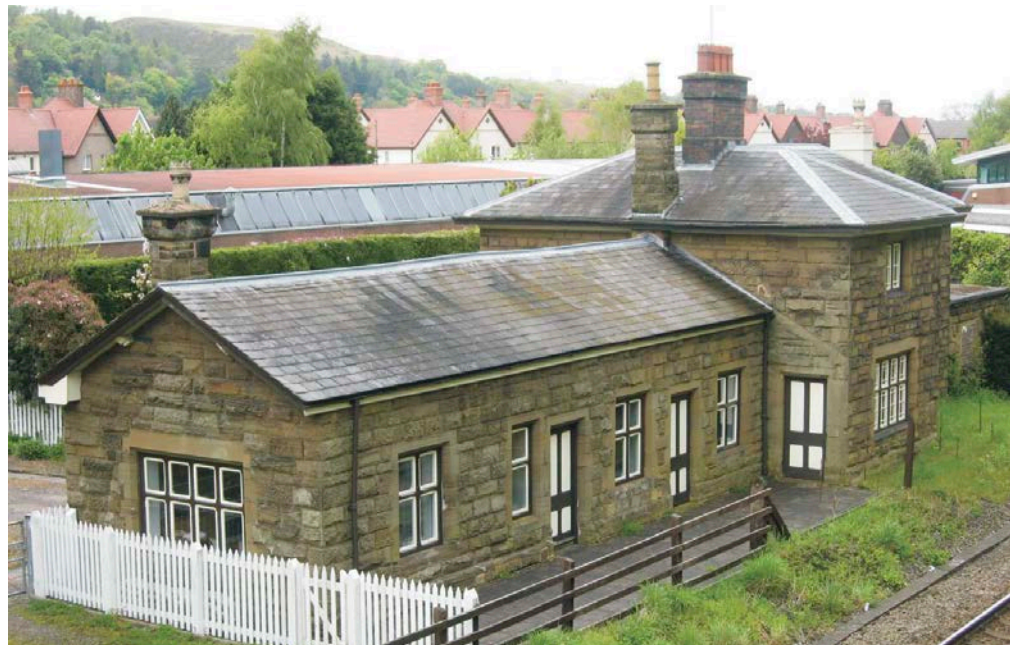
Figure 17: Station house, Church Stretton. Soudley Sandstone.
