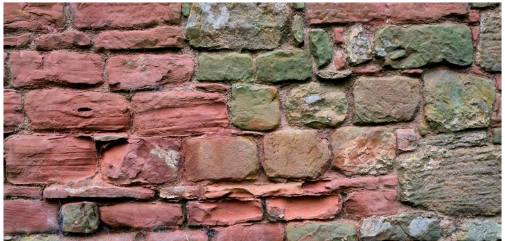
Figure 42: Castle wall, Acton Burnell. Keele Beds sandstone.
