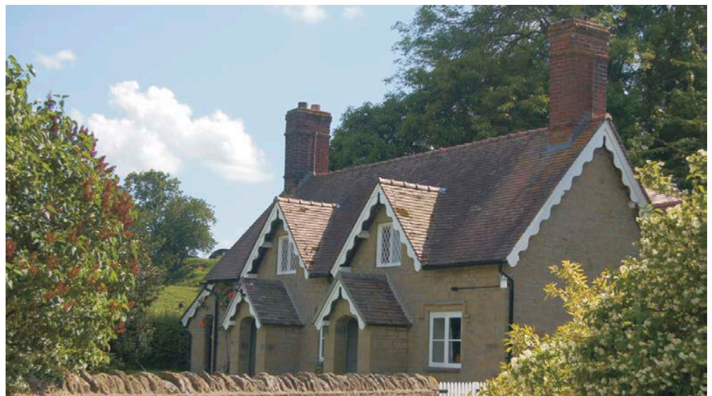
Figure 31: Cottages, Corfton. Downton Castle Sandstone.
