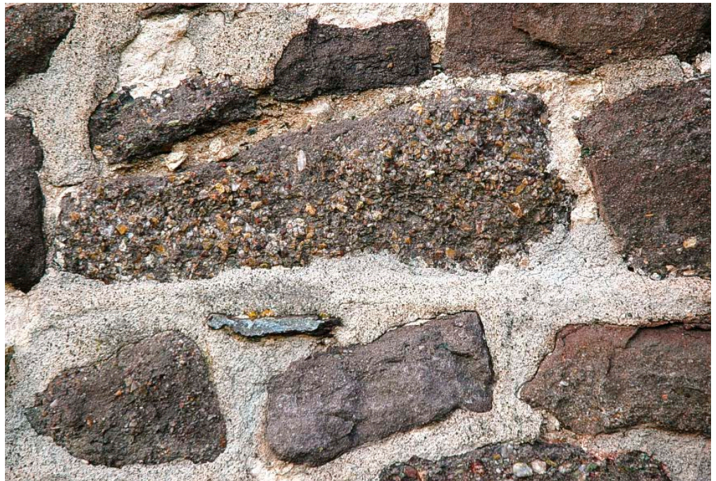
Figure 5: Wall of St Laurence's Church, Church Stretton. Longmyndian conglomerate.
