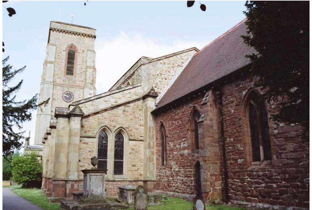
Figure 39: Tower, St George's Church, Pontesbury. Halesowen Formation Sandstone.
