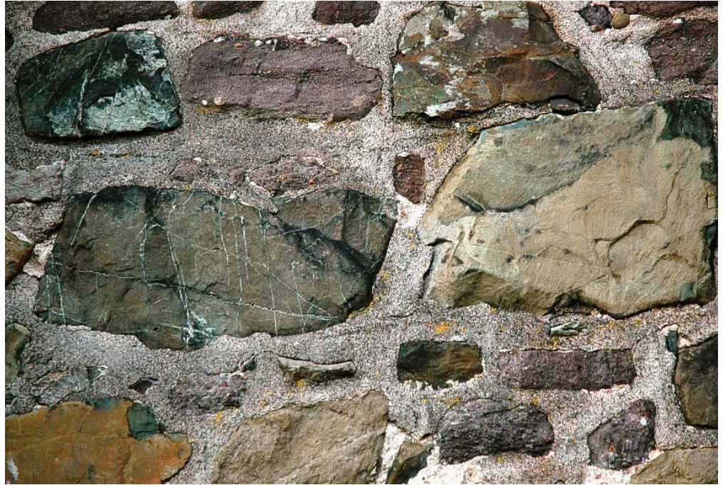
Figure 4: Wall of St Laurence's Church, Church Stretton. Longmyndian stones including fissile mudstones, blocks of Buxton Rock and a boulder of veined dolerite.
