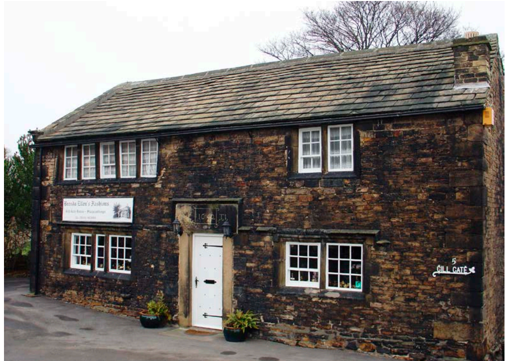
Figure 6: Industrial building with pollution-blackened stonework, Skelmanthorpe.
