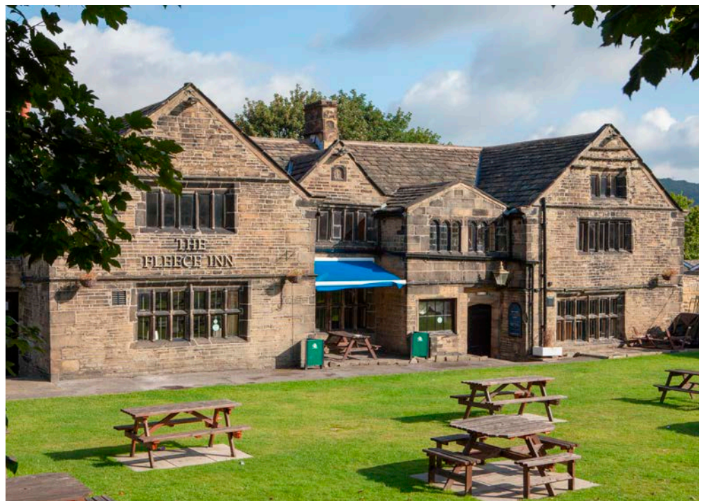
Figure 17: A public house, Elland. Elland Flags and sandstone slate roof.
