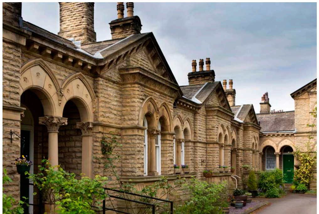
Figure 4: Houses, Saltaire. Millstone Grit.
