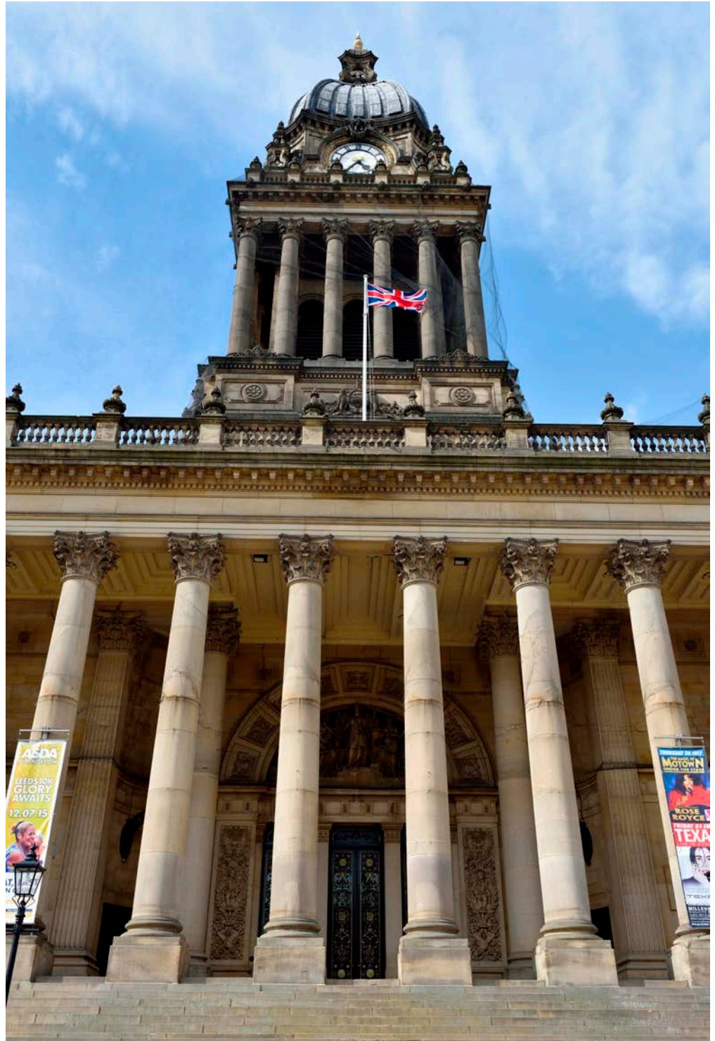
Figure 5: Town Hall, Leeds. Millstone Grit.
