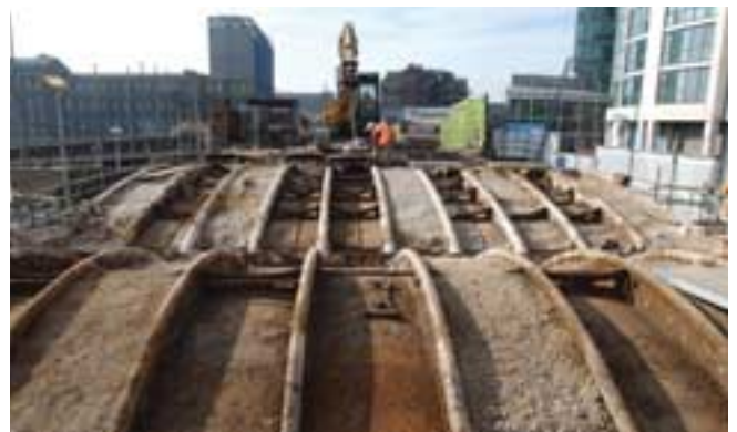
The Brunel bridge being dismantled.
