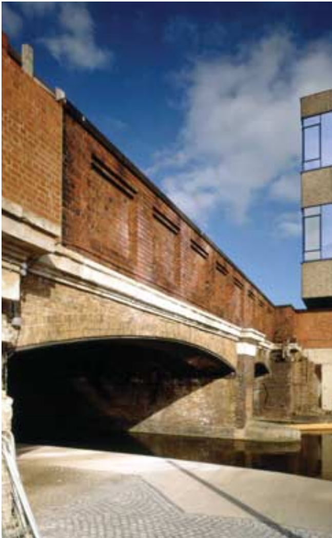
The Bishops Bridge Road bridge concealing Brunel's original structure beneath.
