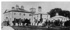
Rokeby Hall, Co. Durham, open as a result of grant aid. (See "Public Access" p2)
