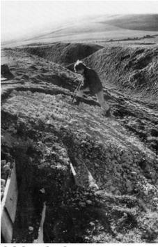
*Work in progress at Barbury Castle, an Iron Age hillfort in Wiltshire, aimed at halting the processes of erosion and re-establishing the profile of the earthworks; measures such as these are sometimes essential for maintaining earthworks under pasture (R Canham, Wilts C C)*
