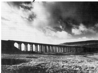
Ribbleshead Viaduct, North Yorks
