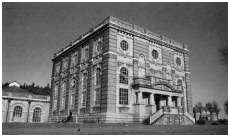
Elkesley Pumping Station: now demolished and the plant scrapped
