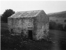
A typical stone barn without its tiles (Y D N P)
