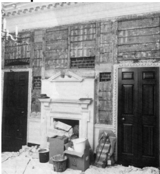
Restoration in progress, Marble Hill
