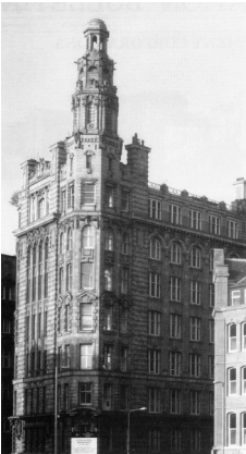
Lancaster House, Whitworth Street, Manchester: a Grade II listed commercial building of 1906, cleaned, repaired, and converted to residential use with grant aid from Central Manchester Development Corporation (CMDC)
