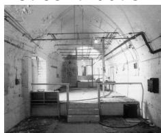
The Hellfire Comer Complex beneath Dover Castle: an operations room
