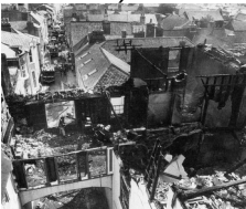
Sifting the debris after the Totnes fire: the fire spread rapidly through the undivided roof spaces in the building flanking the archway (Herald Express)
