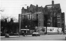
The Belgrave Hospital, Clapham Road, Lambeth: an early twentieth-century disused hospital under active consideration for hostel use for the homeless
